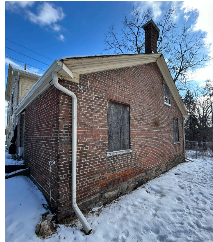
Tail wing and its double-wythe red brick cladding (ERA, 2025)
