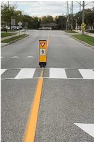
Flexible Bollard at PXO
