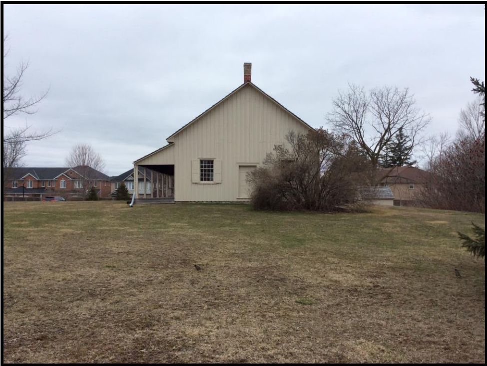
Image 26: View of East Elevation of Orthodox Friends Meeting House (Photo taken on April 7, 2016, Facing West)
