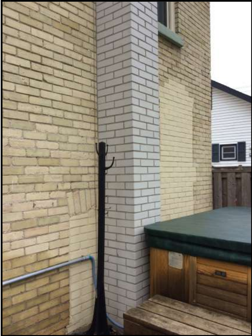
Image 7: North Elevation Showing Filled Door and Window Openings and Chimney Addition (Photo taken on April 7, 2016; Facing Southwest)
