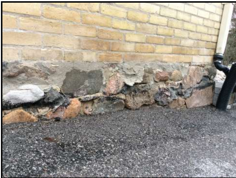
Image 4: Stone Foundation, West Elevation (Photo taken on April 7, 2016; Facing Southeast)
