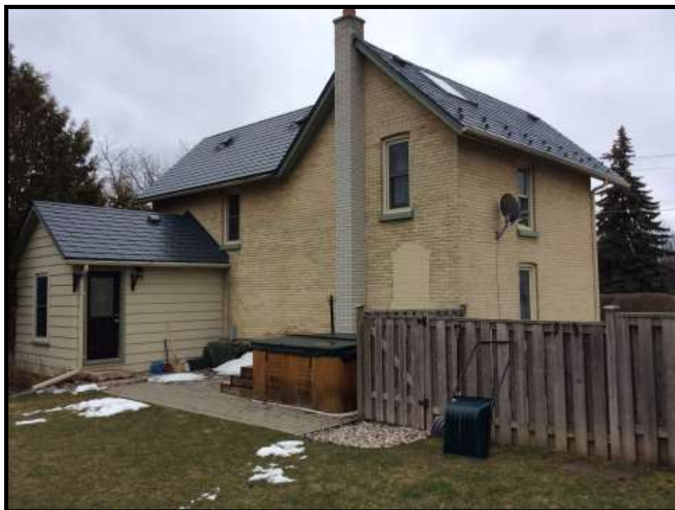
Image 6: North Elevation of 411 Millard Avenue (Photo taken on April 7, 2016; Facing Southeast)
