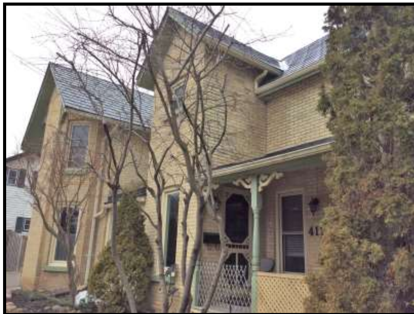
Image 2: Detail of Façade (Photo taken on April 7, 2016; Facing Northwest)
