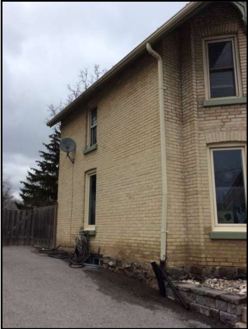
Image 5: West Elevation of 411 Millard Avenue (Photo taken on April 7, 2016; Facing Northeast)
