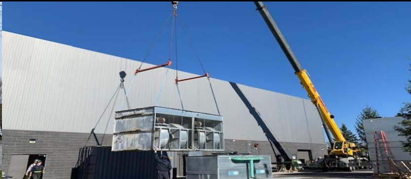
Replacement at Facilities
