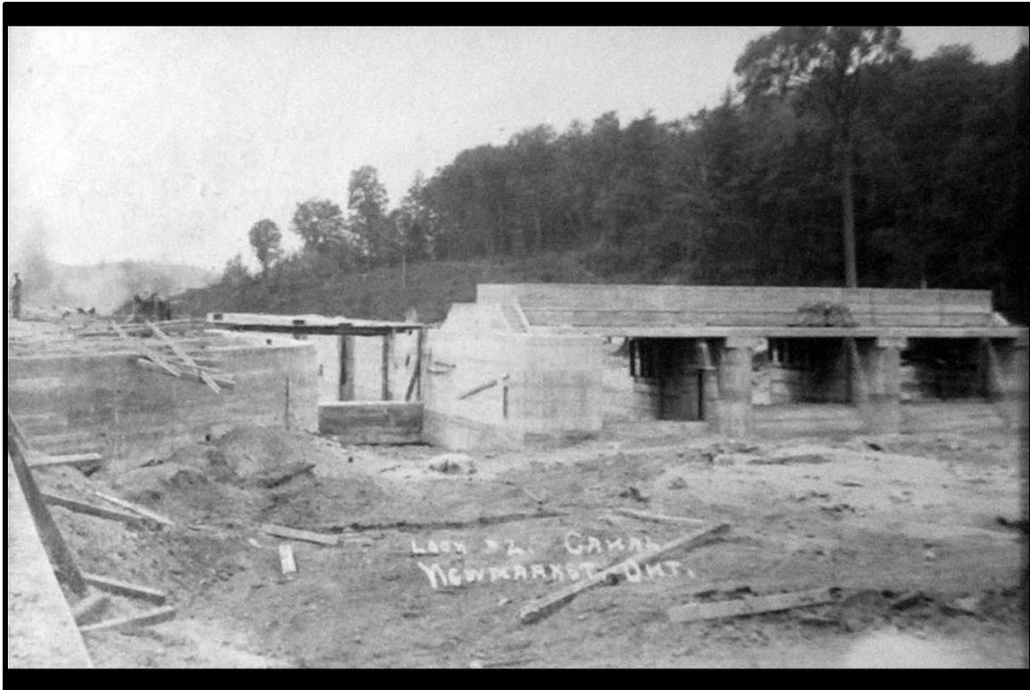
**Plate 3: Construction of Lock 2**
