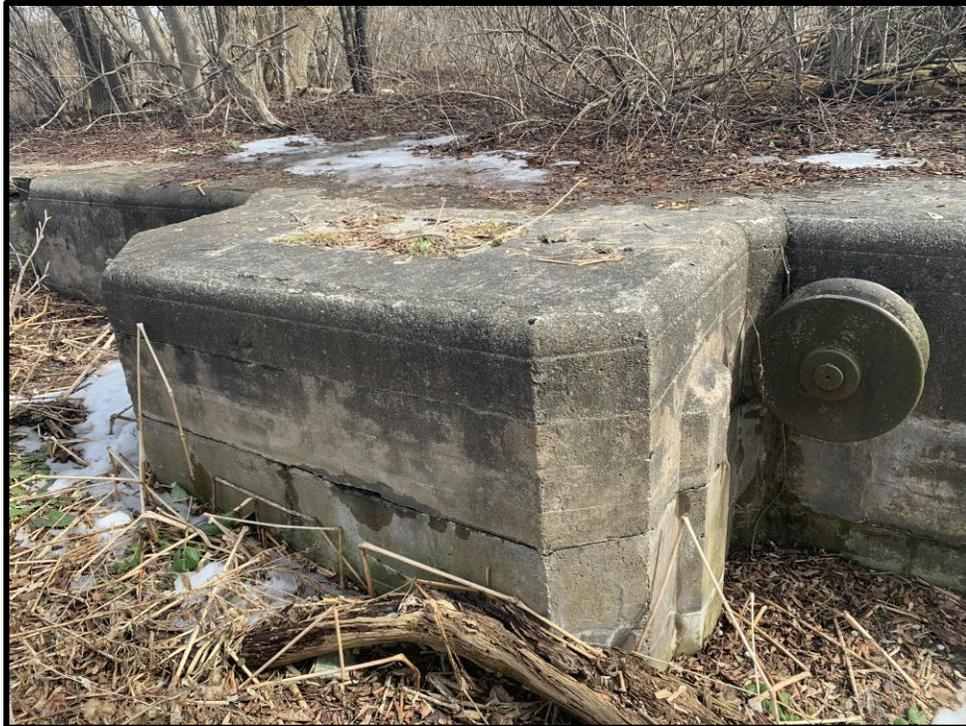
**Image 18: Detail of pulley system south side of Lock 3
