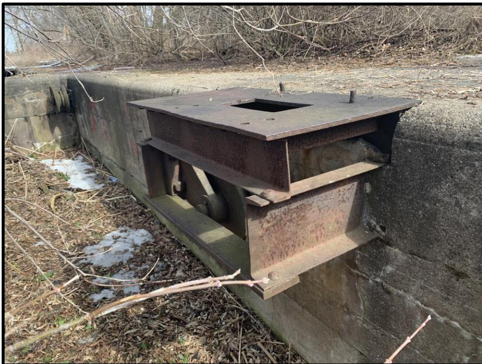
**Image 17: Pulley system south side of Lock 3**
