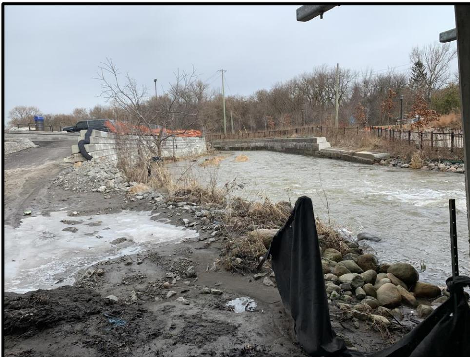
**Image 33: Original poured-in-place concrete canal east wall with recent stepped cuts**
