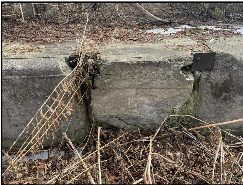
**Image 15: Detail of board marks in concrete of Lock 3
