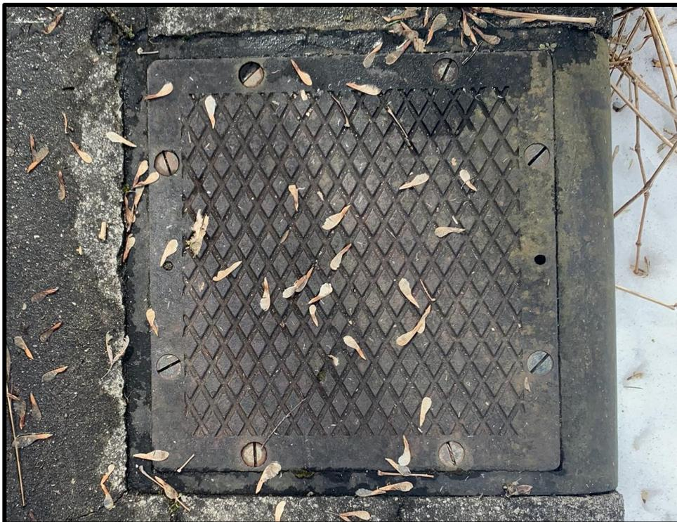
**Image 13: Access panel to drain lock chamber of Lock 3
