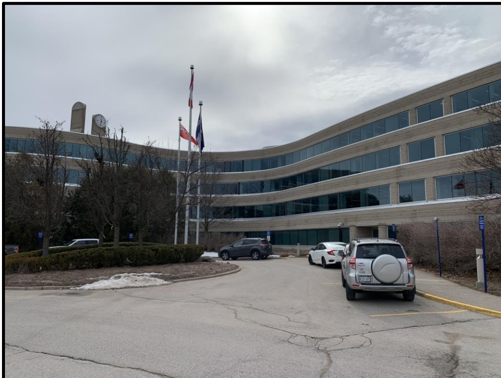
Image 21: Parking lot (north) side circular driveway (Photo taken on March 11, 2020; Facing Southeast)
