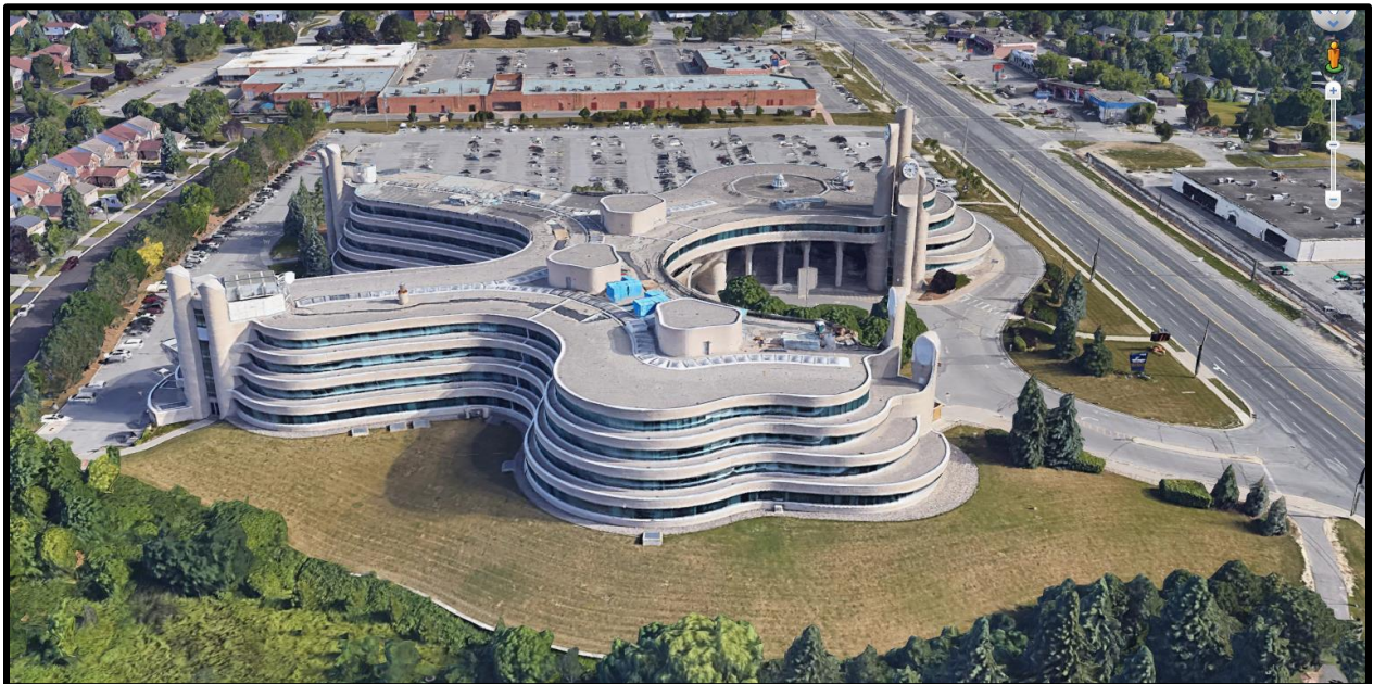
Figure 2: Oblique view of 17250 Yonge Street looking north (Google Earth 2005; Facing North)
