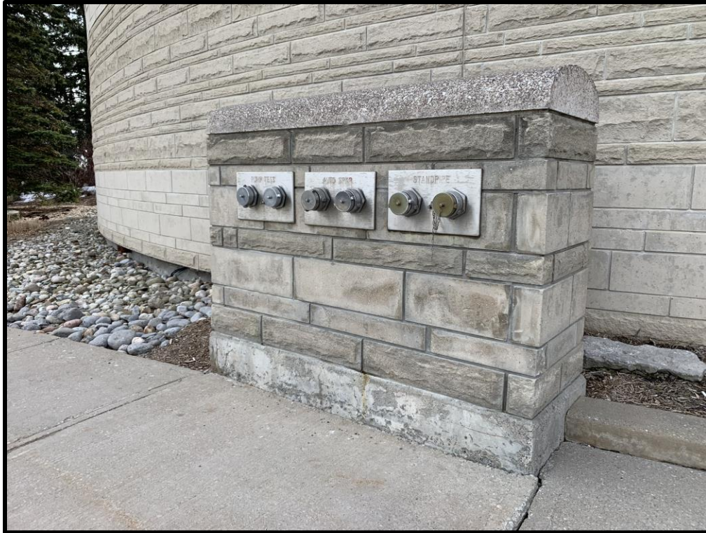
Image 24: Sympathetically designed and constructed water hook up (Photo taken on March 11, 2020; Facing Southeast)
