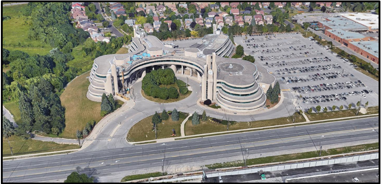
Figure 1: Oblique view of 17250 Yonge Street looking west (Google Earth 2005; Facing West)
