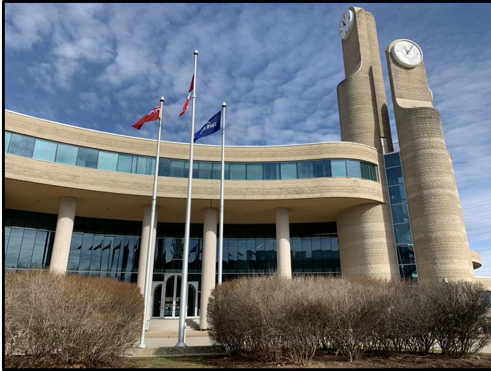
Image 1: Main entryway – Northeast wing (Photo taken on March 11, 2020; Facing North)
