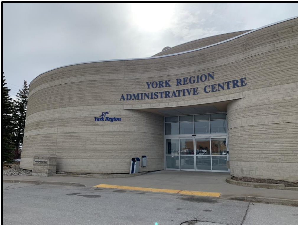
Image 23: Parking lot entryway, north side (Photo taken on March 11, 2020; Facing Southeast)
