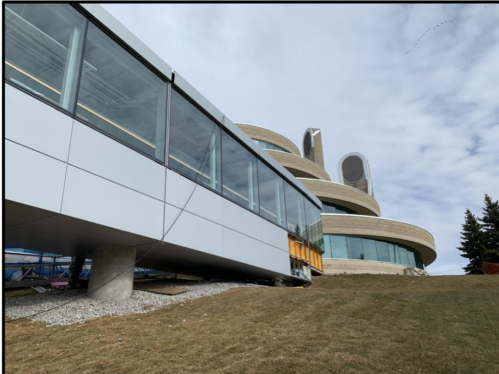
Image 12: Enclosed walkway access looking toward southeast wing (Photo taken on March 11, 2020; Facing West)
