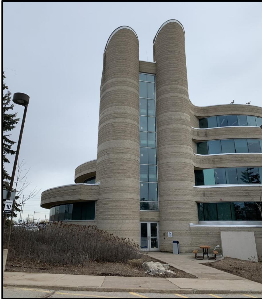
Image 19: Secondary entryway between northwest towers (Photo taken on March 11, 2020; Facing East)
