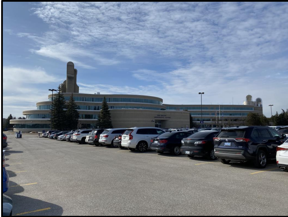
Image 26: North side – Northeast wing with four clock towers (left) and northwest wing, each with two towers (Photo taken on March 11, 2020; Facing East)
