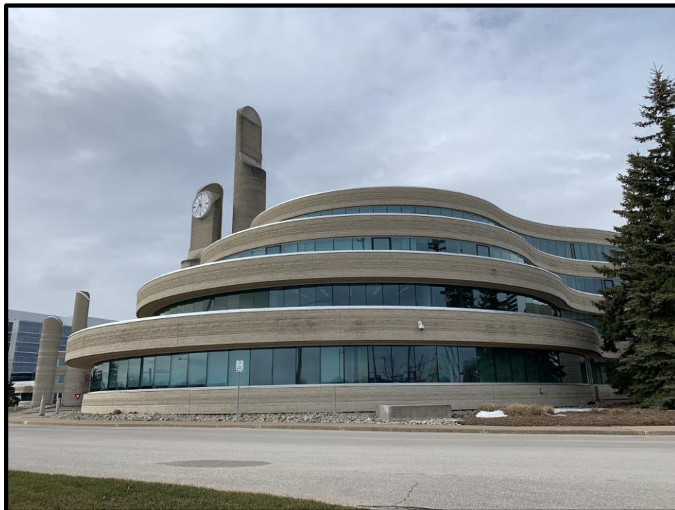
Image 27: Northeast wing with clock towers (Photo taken on March 11, 2020; Facing southwest)
