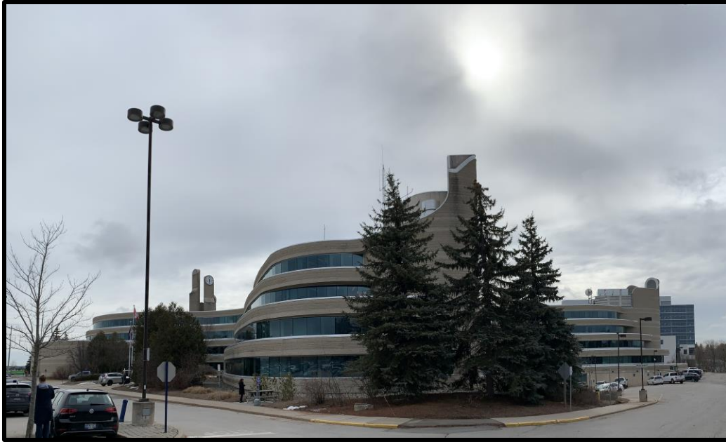
Image 20: Northwest wing (Photo taken on March 11, 2020; Facing Southeast)
