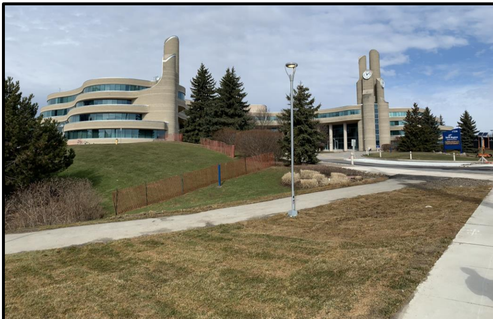
Image 6: View to main entryway from Yonge Street (Photo taken on March 11, 2020; Facing Northwest)
