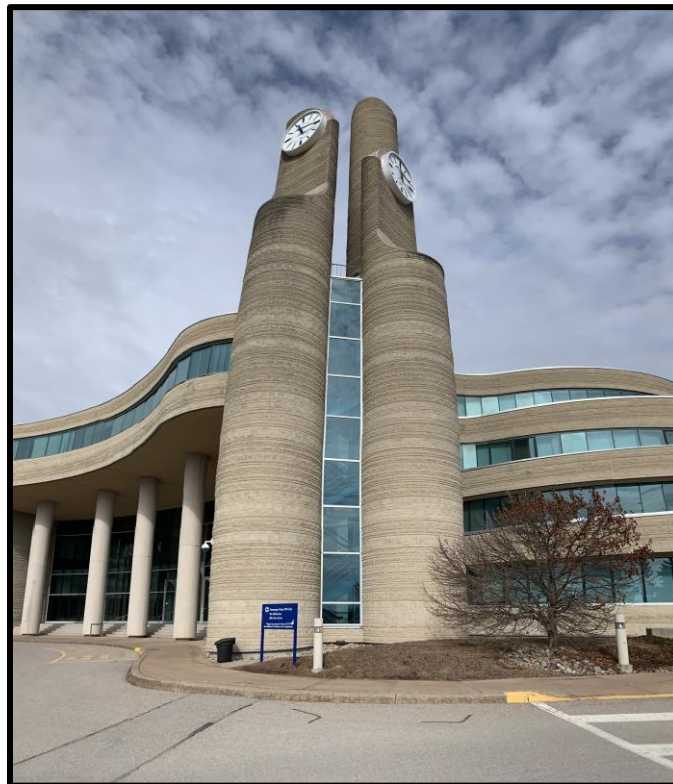
Image 4: Four clock towers – Northeast wing (Photo taken on March 11, 2020; Facing Northwest)
