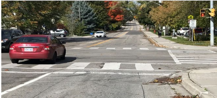
Lorne Avenue Reconstruction
