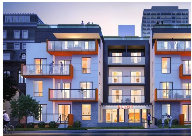
Recesses, projections, materials and balconies break these buildings into smaller components visually.
