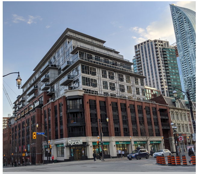
Vertical articulation used to break buildings into smaller components that reflect existing tight-knit retail streets.
