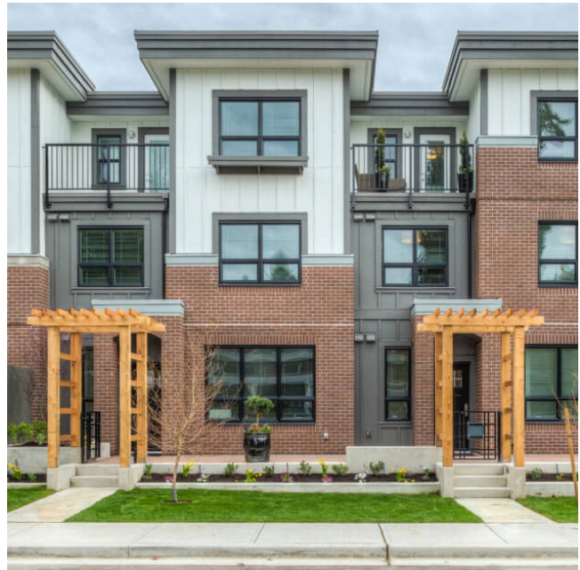
Recesses and projections create vertical articulation, while materials are used to define horizontal scale.
