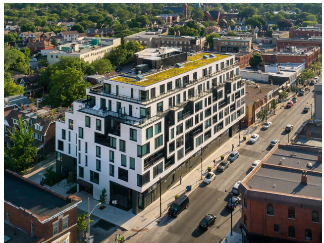
A rear-angular plane used to inform the mass of the building and provide a transition to adjacent dwellings.
