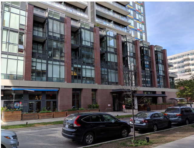
Top: Narrow towers minimize shadow impacts. Bottom: A human-scaled podium anchors the tower.
