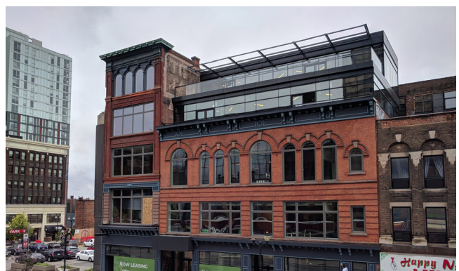
Stepbacks are used to provide transitions to adjacent properties and to mitigate shadows impacts.
