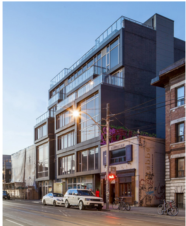
Podiums can be used to reinforce an established streetwall while providing private patio space.
