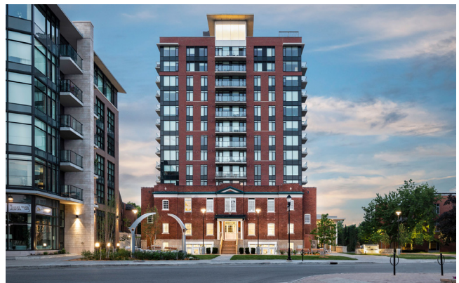
The height of a high-rise building should clearly relate to adjacent buildings.
