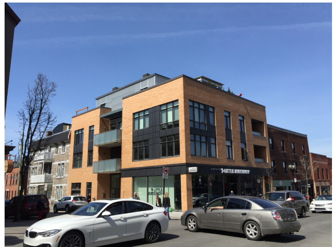
Mid-rise buildings should be massed to respond to their adjacent and established context.
