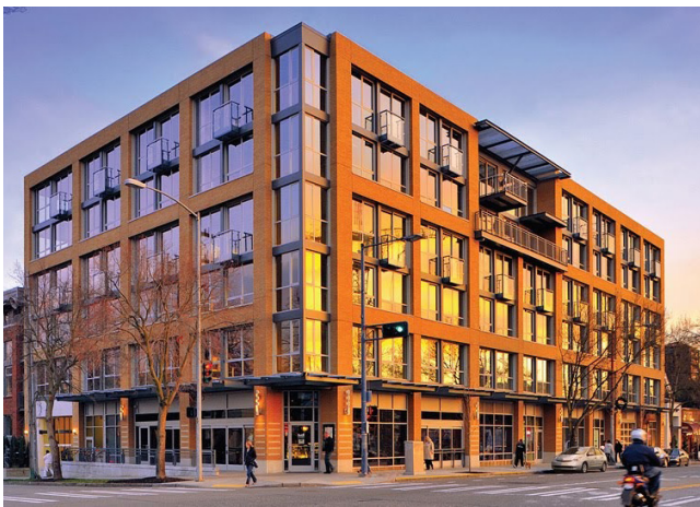
Clear podiums (top) and vertical articulation (bottom) used to define a human-scale in larger buildings.
