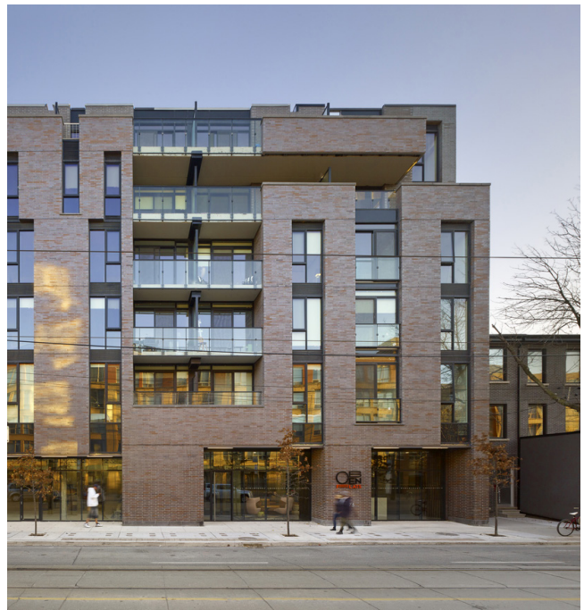
Side-yard setbacks, materials and window alignment used to create a strong transition to adjacent uses.
