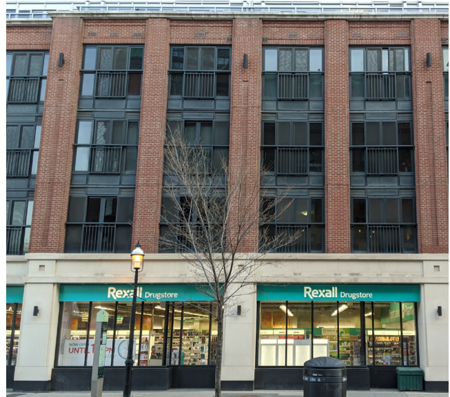
Large, highly transparent grade-level windows enhance safety and provide opportunities for casual surveillance.
