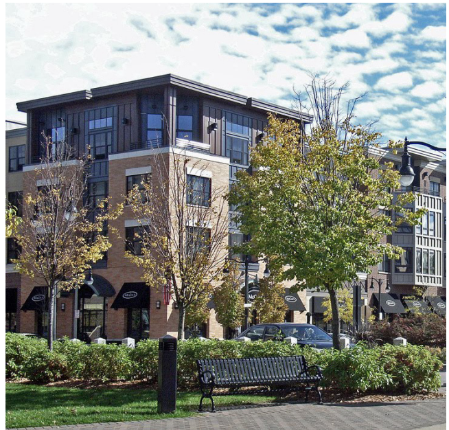
Stepbacks at the upper levels of a building help to mitigate shadows on adjacent streetscapes and parks.
