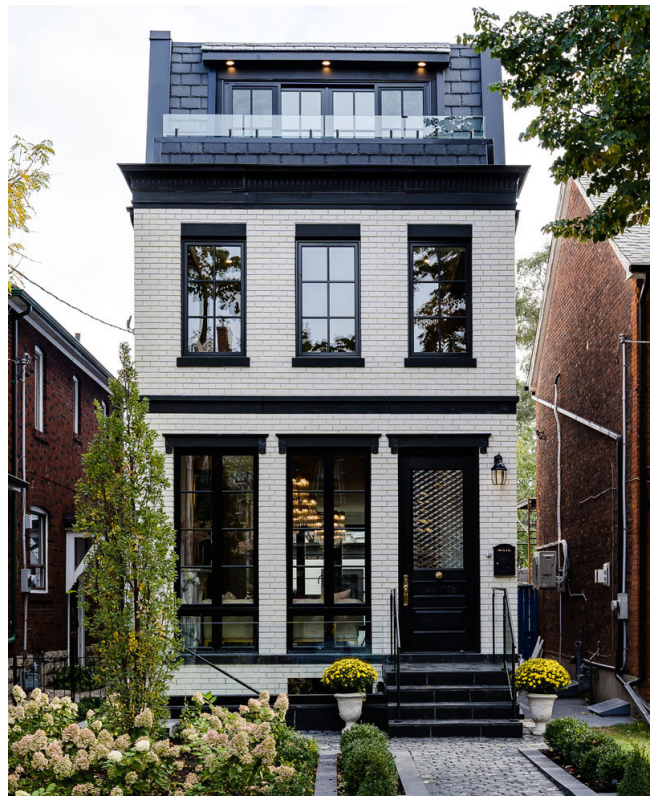
Well-spaced, human-scaled building with clearly articulated entrances, levels and upper storeys.
