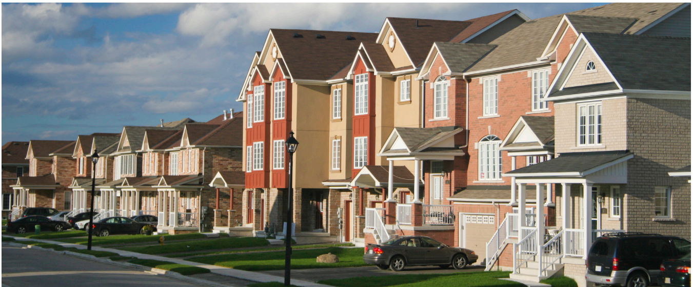
Consistent, but varied, materials help to create an attractive streetscape.
