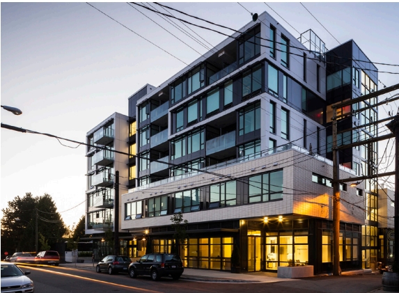
Ensure safety and accessibility for all
