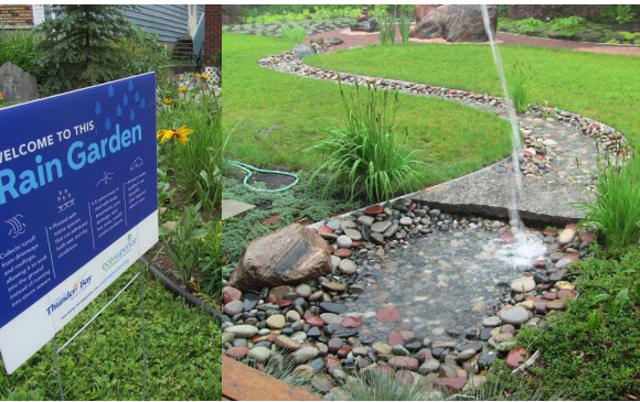
Left: Rain garden showing aggregate surfaces for infiltration and plantings, Right: soakaway trench combined with a high downspout
