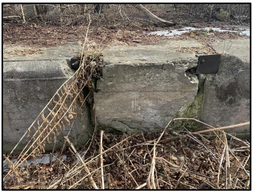
Image 15: Detail of board marks in concrete of Lock 3 (Photo taken on March 11, 2020: Facing West)
