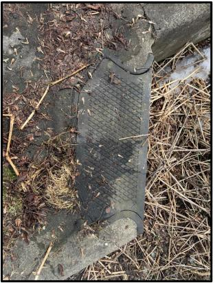
Image 14: Access panel to drain south end of lock chamber Lock 3 (Photo taken on March 11, 2020)
