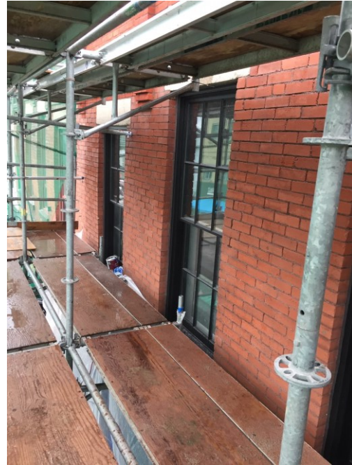
Photo 5: Restored front facade at 194 Main Street
