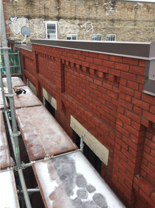
Photo 4: Restored parapet at 194 Main Street
