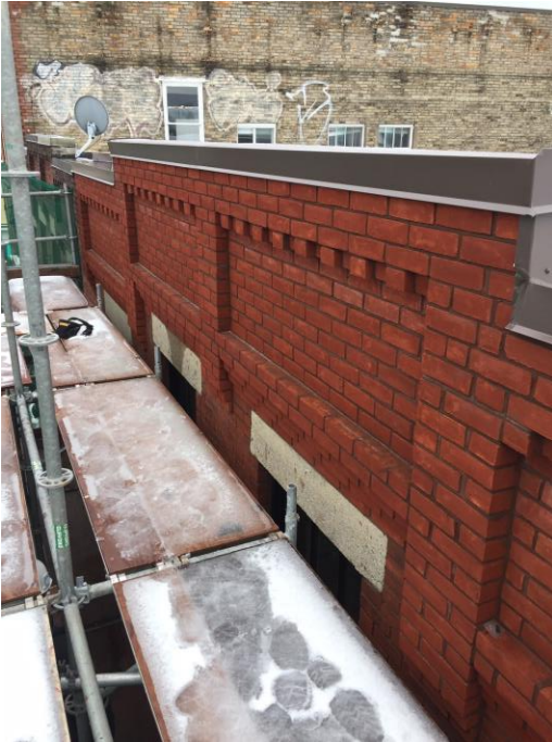
Photo 4: Restored parapet at 194 Main Street
