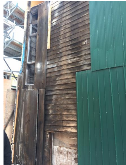
Photo 2: North elevation of 188 Main Street
