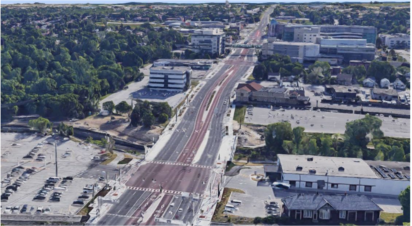
Figure 8. View at Davis Drive and GO Rail Corridor
