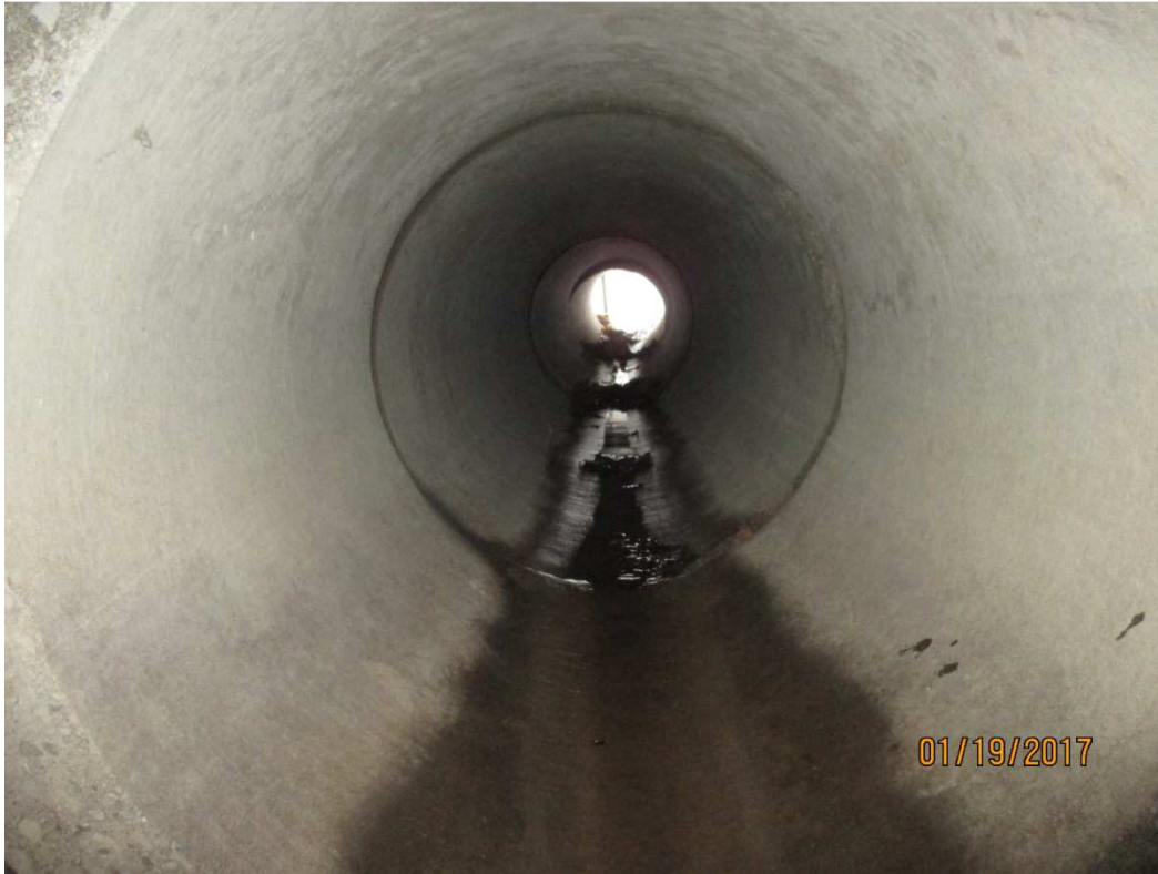
Photo 7 – Looking Up Storm Pipe Penetration – Note Displaced Pipe Segments
