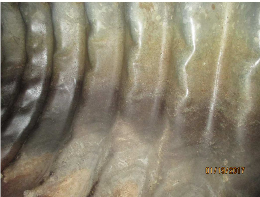
Photo 12 – Medium to Severe Crimping of Section 2 of East Culvert Pipe
