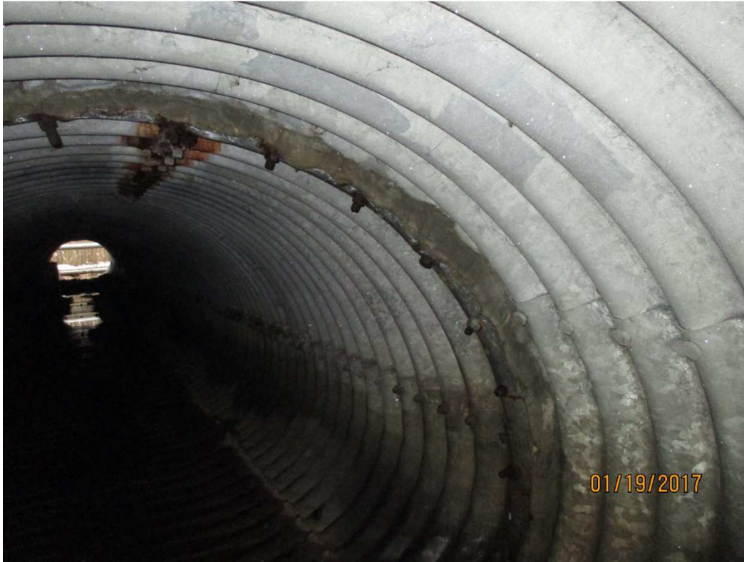
Photo 17 – Connection between Section 2 and Section 3 of East Culvert Pipe
