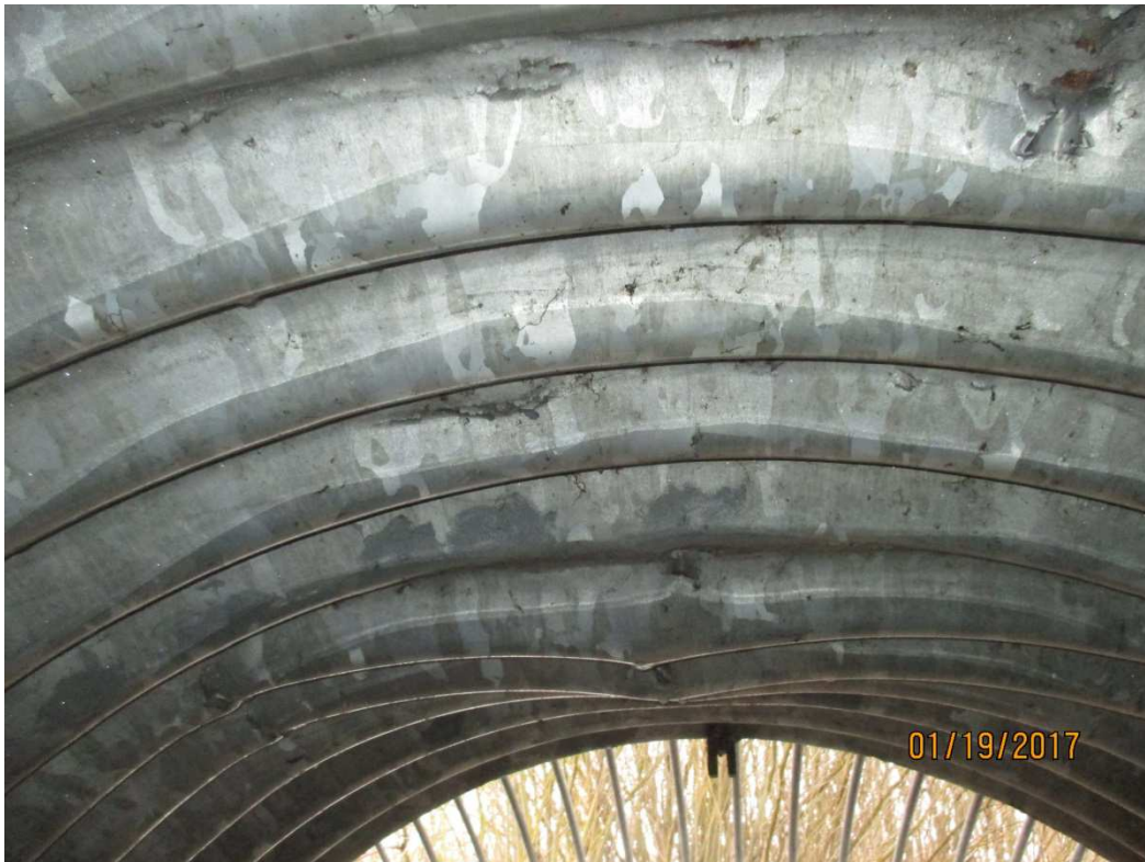
Photo 8 – Deformation of Culvert Soffit near Inlet
