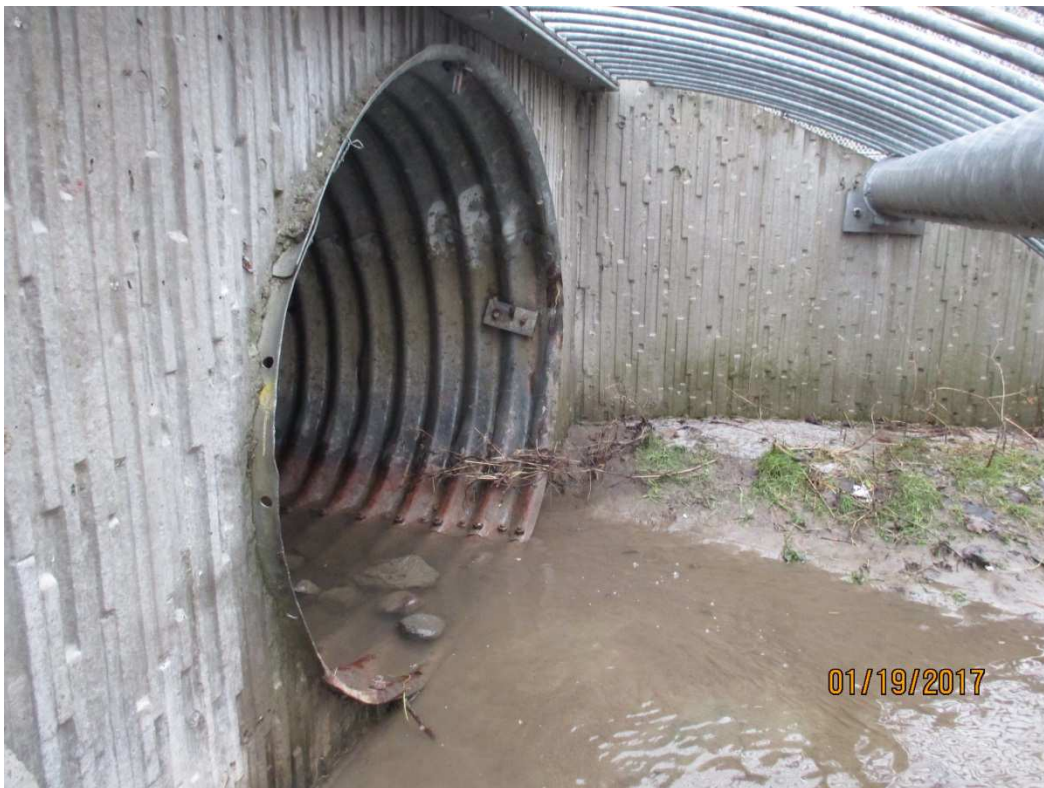
Photo 4 – Inlet of East Culvert Pipe – Multi Plate Corrugated Steel Pipe Arch
