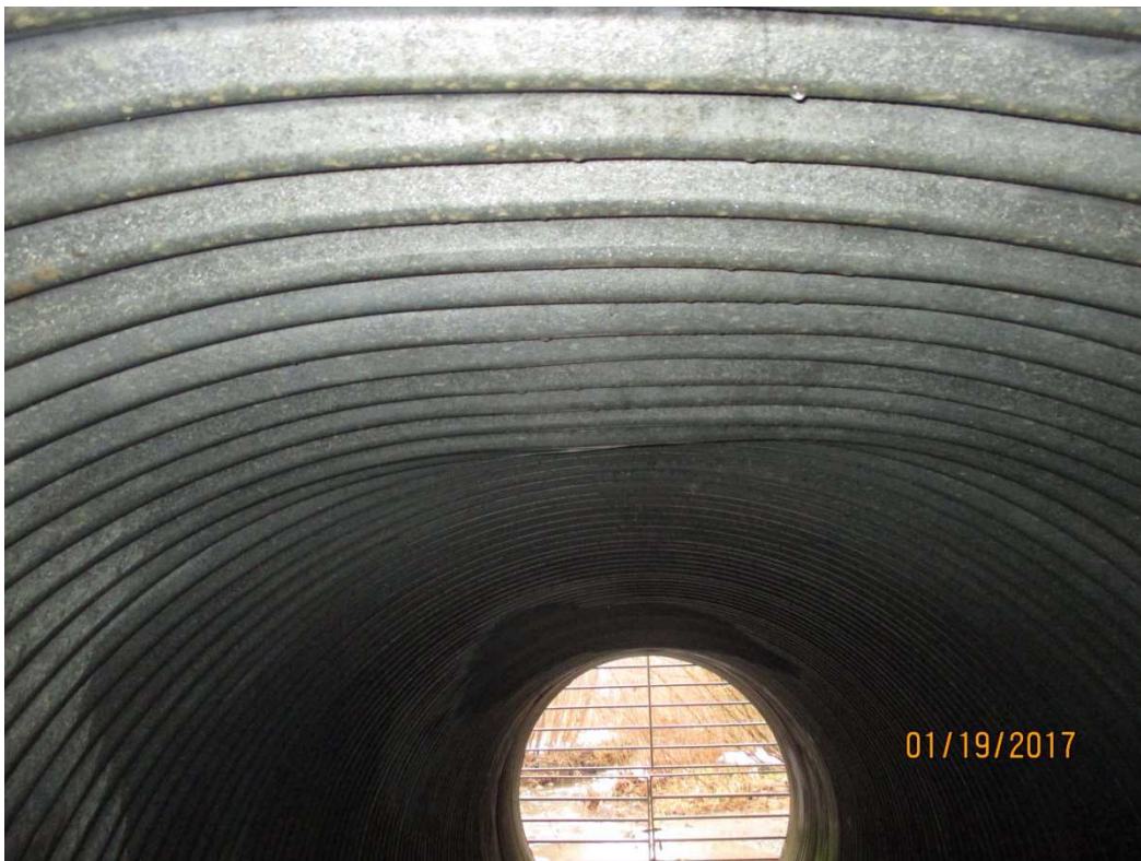
Photo 24 – Deformation of Culvert Obvert at Outlet of East Culvert Pipe
