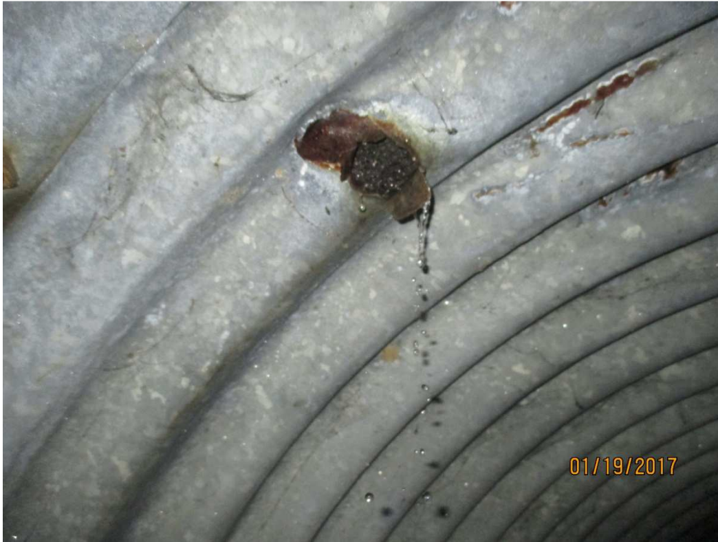
Photo 15 – Perforation & Leakage of Section 2 of East Culvert Pipe
