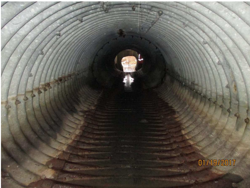
Photo 10 –Section 2 of East Culvert Pipe – Multi Plate CSPA Looking Towards Outlet
