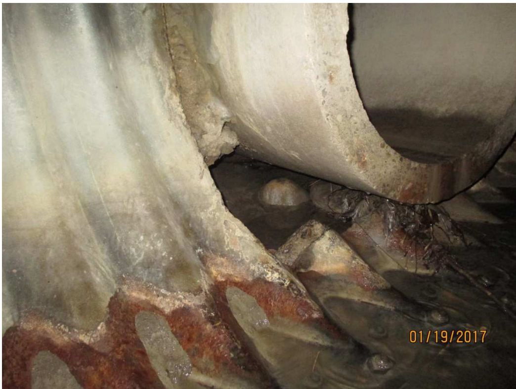
Photo 6 – Oversized Cut and Missing Parging at Storm Pipe Penetration
