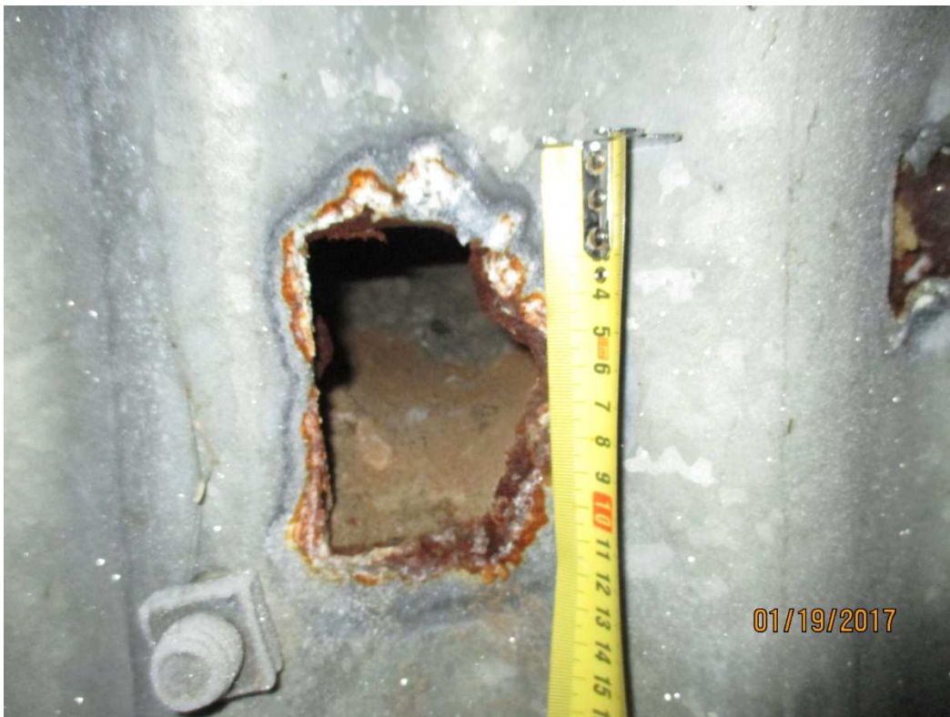
Photo 14 – Perforation of Section 2 of East Culvert Pipe
