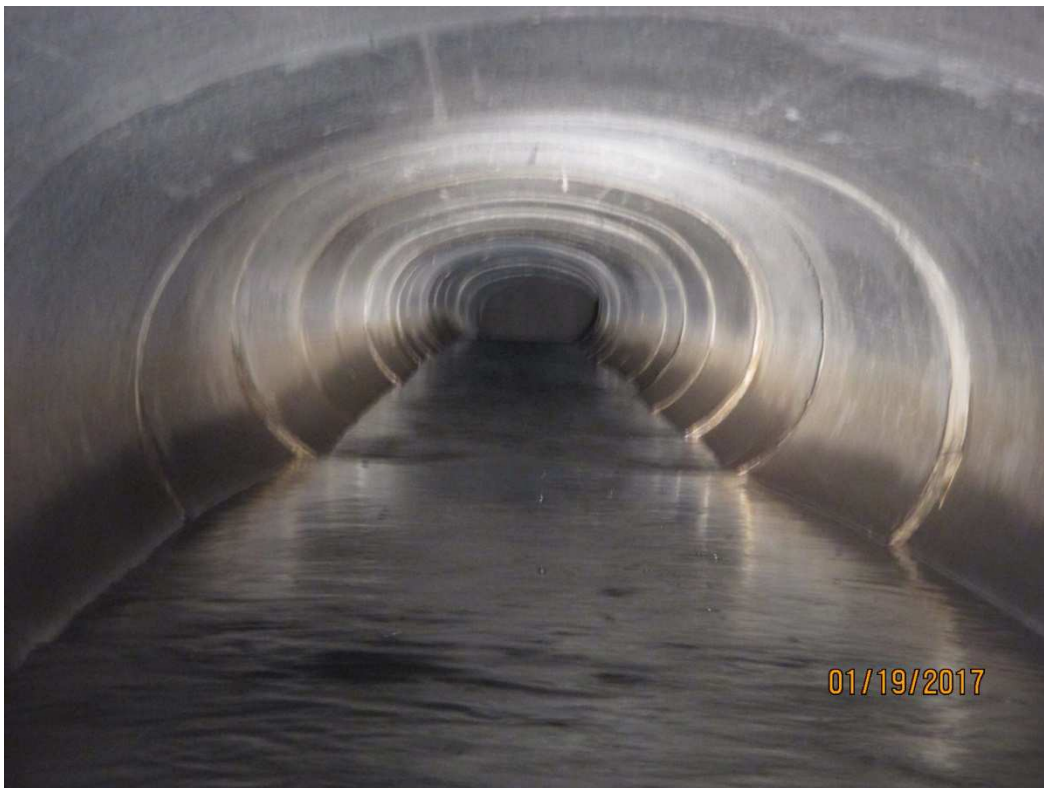
Photo 2 – West Pipe (Concrete Ellipse) Looking Downstream
