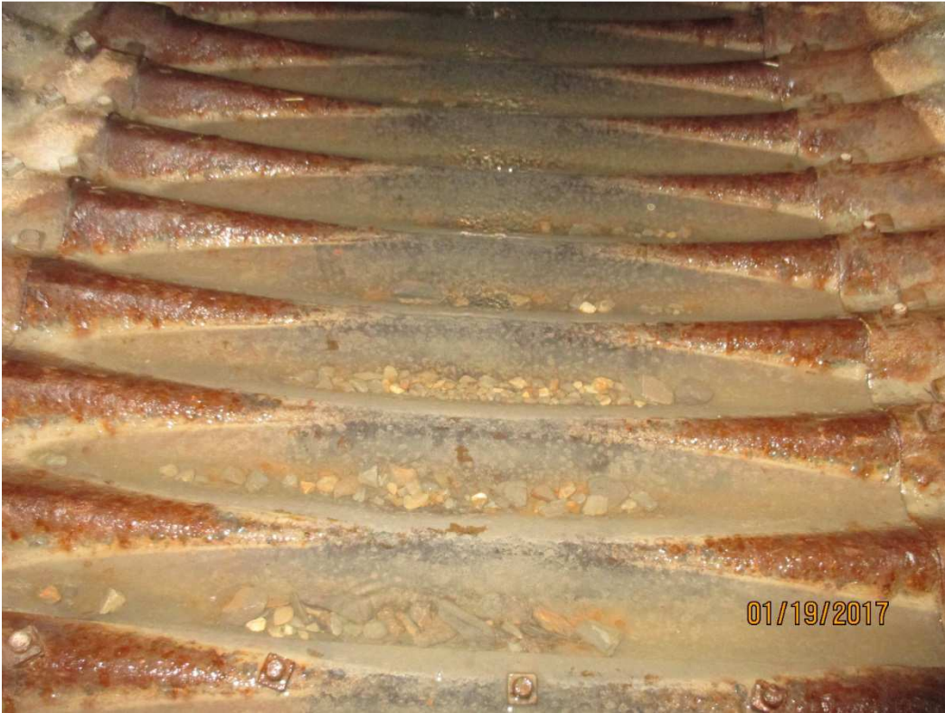
Photo 11 –Corrosion of Section 2 of East Culvert Pipe Invert
