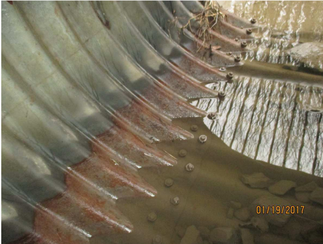
Photo 5 –Corrosion of Culvert Invert near Inlet
