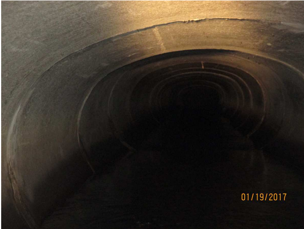
Photo 3 – West Pipe (Concrete Ellipse) Displaced Pipe Segment
