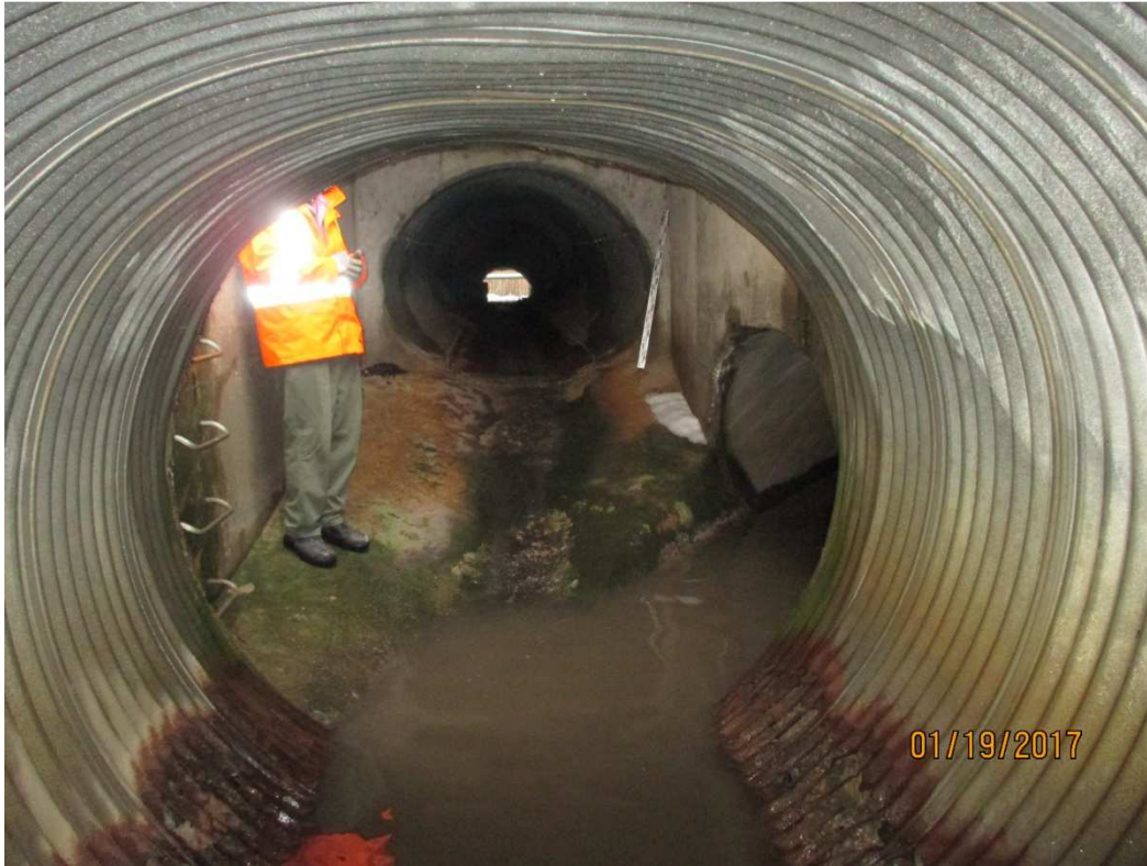
Photo 19 – Concrete Drop Maintenance Hole Structure Looking from Section 4 (Outlet) of East Culvert Pipe
