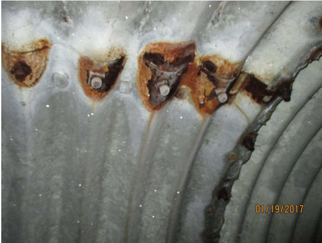
Photo 13 – Corrosion of Bolt Connections of Section 2 of East Culvert Pipe
