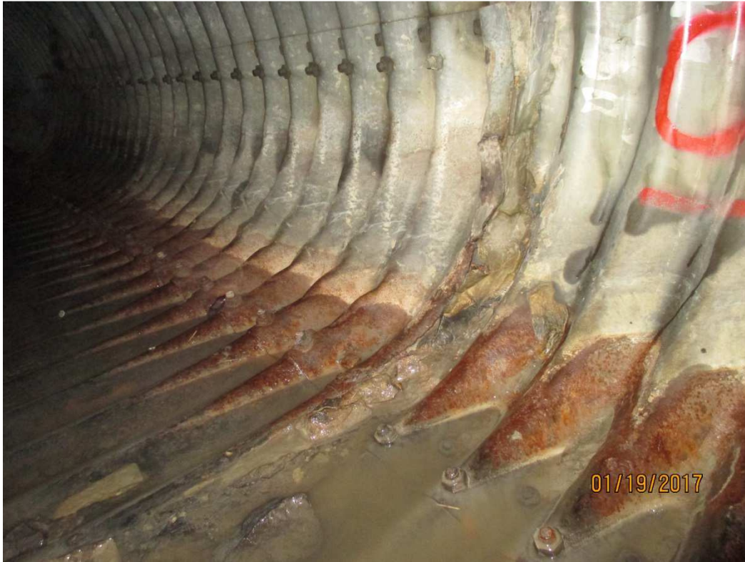
Photo 9 – Connection between Section 1 and Section 2 of East Culvert Pipe
