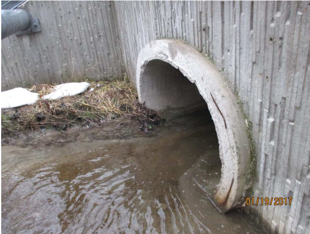
Photo 1 – Inlet of West Culvert Pipe - Concrete Ellipse
