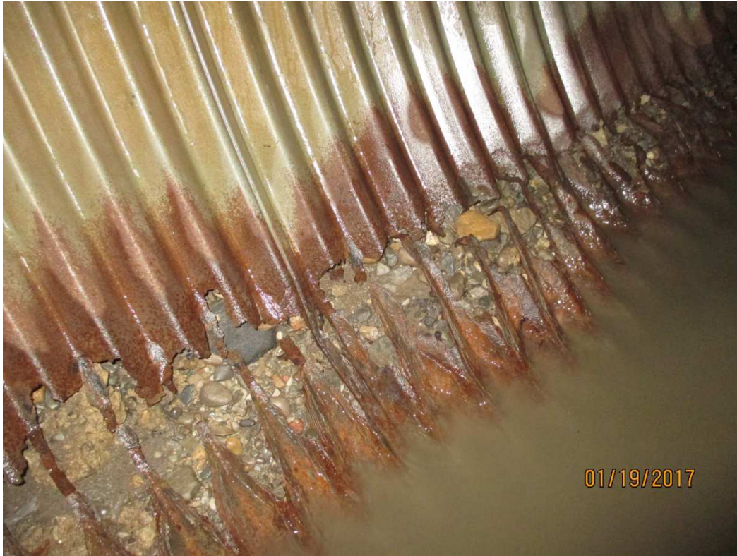
Photo 23 – Corrosion with Critical Perforations & Section Loss – West Side of Section 4 of East Culvert Pipe
