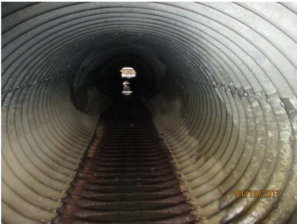
Photo 16 –Section 3 of East Culvert Pipe – Multi Plate CPSA Looking Towards Inlet
