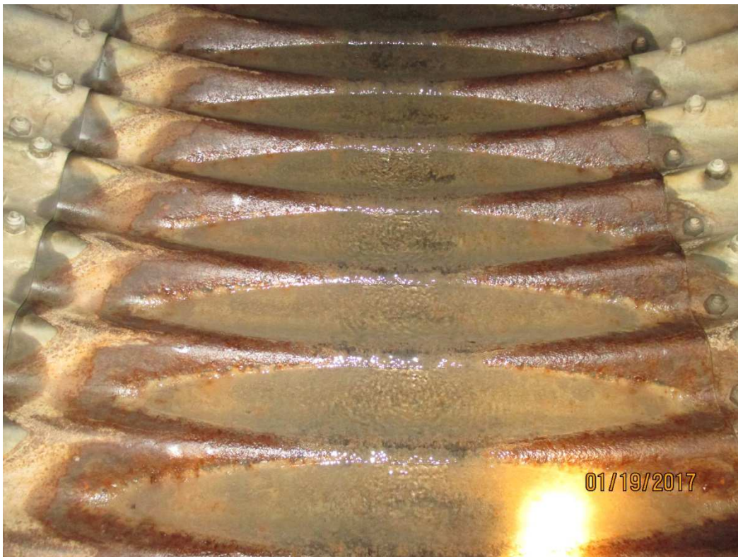
Photo 18 –Corrosion of Section 3 of East Culvert Pipe
