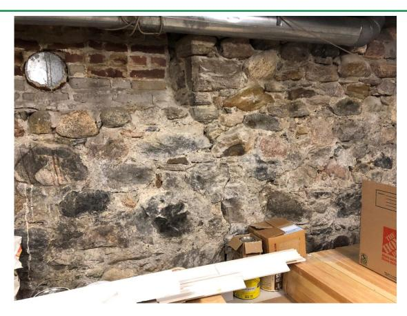
Photo 2 - Existing field-stone rubble foundation wall with evidence of efflorescence stains and vertical crack extending from previous window opening.
