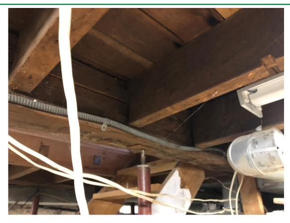
Photo 3 - Existing framing for ground floor and mortise and tenon joint into main structural beam.
