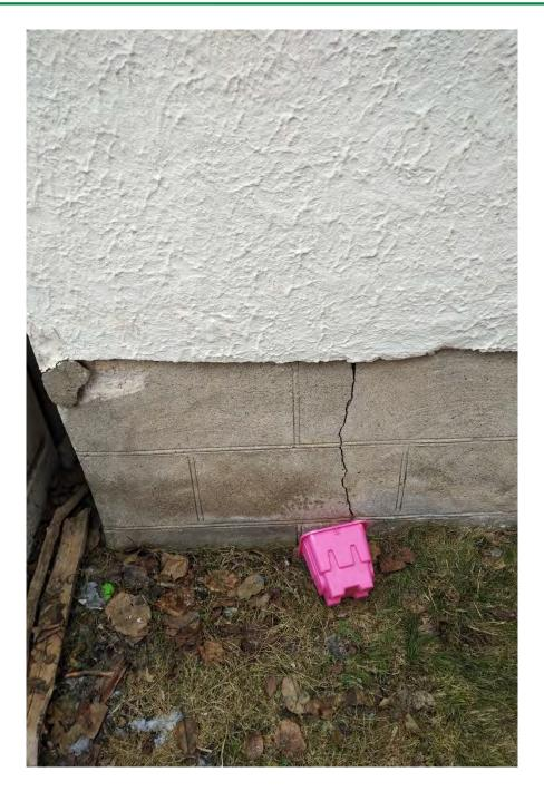
Photo 6 – Large vertical crack in north foundation wall (172 Victoria St)
