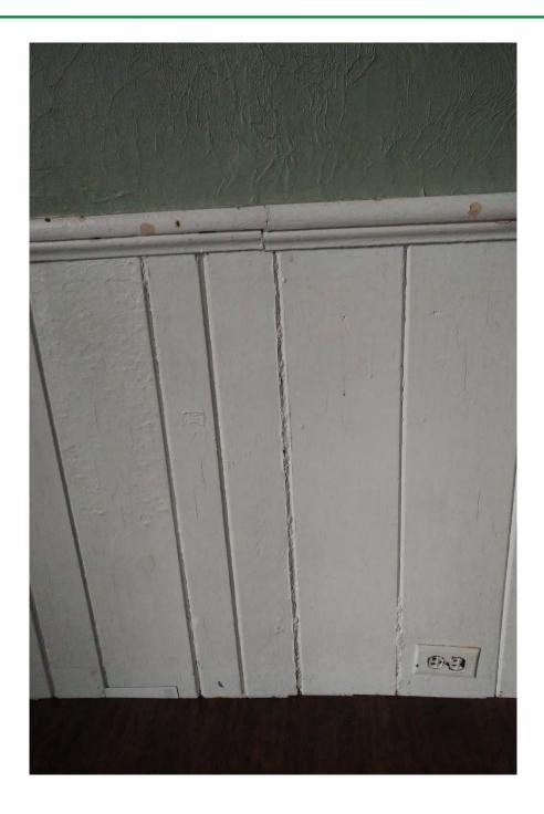
Photo 22 - Typical crack in wall finishes at ground floor (174 Victoria St).
