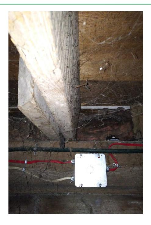
Photo 18 – Example of twisting and notching at ends of joist at party wall
