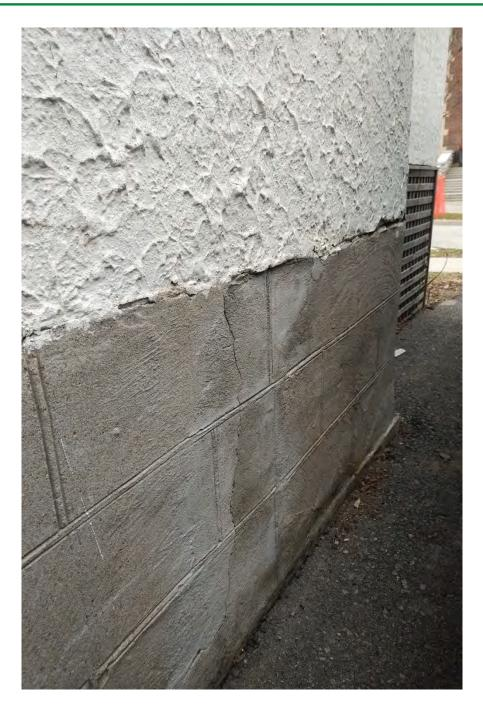
Photo 4 – Vertical crack in south foundation wall
