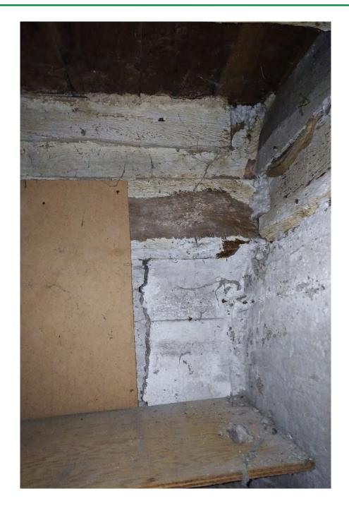
Photo 17 – Vertical crack in interior of foundation wall (174 Victoria St).
