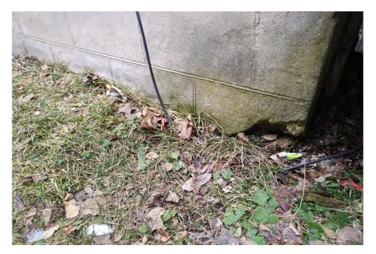
Photo 8 – Material loss in northwest corner of foundation wall (172 Victoria Street)
