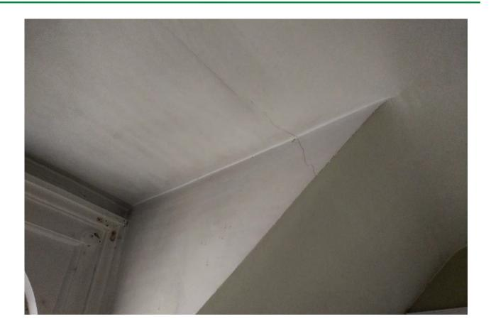
Photo 23 – Sample crack in ceiling finishes at second floor.
