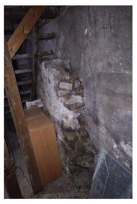
Photo 16 – Section of original rubble wall – no longer loadbearing (174 Victoria St)
