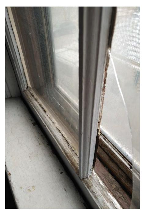
Photo 24 - Typical condition of window frames (174 Victoria St).
