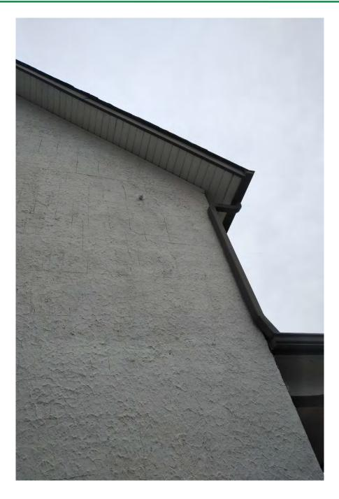
Photo 5 - Typical cracking in stucco finish evident across entirety of south elevation (174 Victoria St)
