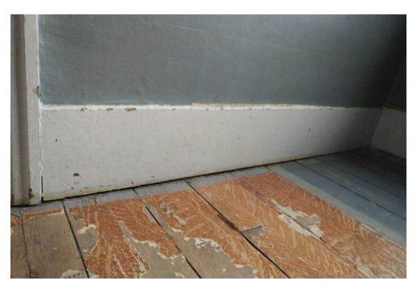
Photo 20 – Gap between base board and first floor planks
