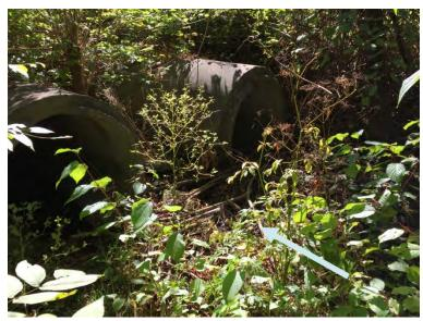
Photo 5: Entrance to concrete pipe culverts under GO Transit rail line
