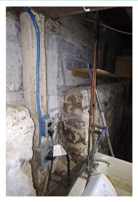
Photo 14 – Front end post, noted to be rotting at base (174 Victoria St)
