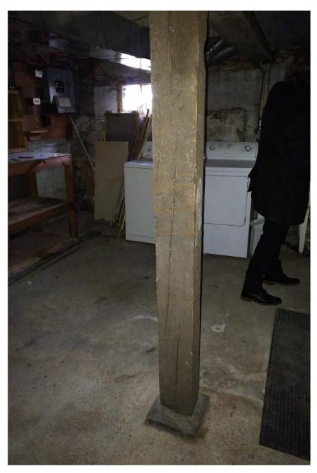
Photo 11 – Interior wood post, on mud sill, exhibiting vertical splitting (174 Victoria St)
