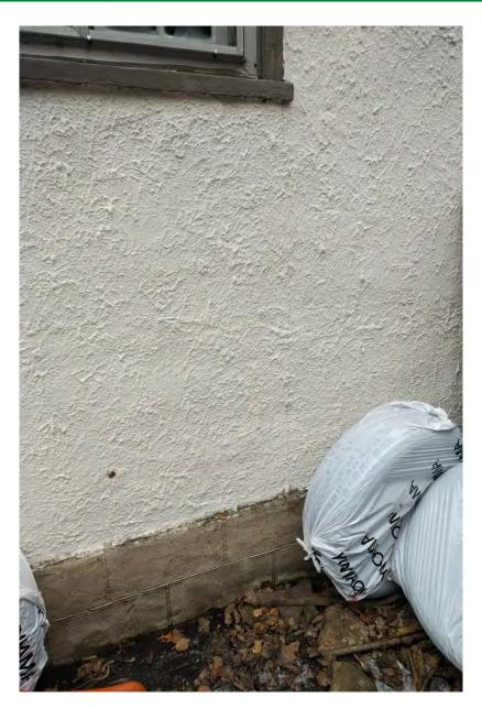
Photo 9 – Vertical crack in stucco finish, and in block foundation wall (172 Victoria Street)
