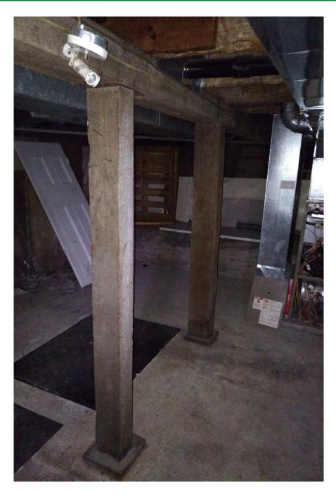
Photo 10 – Central wood beam, supported by timber posts on wood sills in basement (174 Victoria St)
