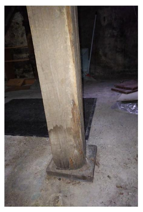
Photo 12 – Interior wood post, on mud sill, exhibiting rotting at base (174 Victoria St)
