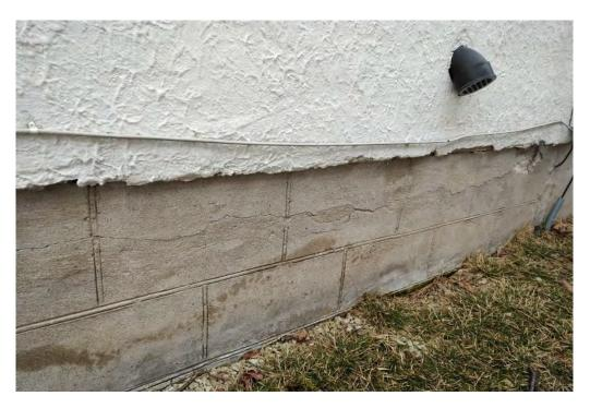
Photo 7 – Horizontal crack in north foundation wall (172 Victoria Street)
