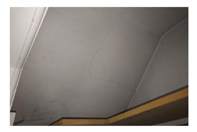
Photo 21 - Typical crack in ceiling finish. Note that this a representation of typical crack patterns, frequency and size within the entire unit (174 Victoria St).
