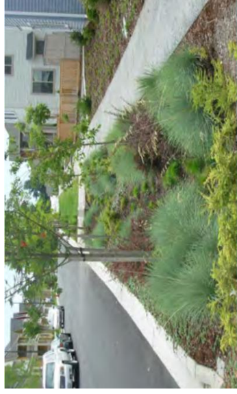
Bioretention Swale – "Grey to Green Road Retrofits", Credit Valley Conservation
