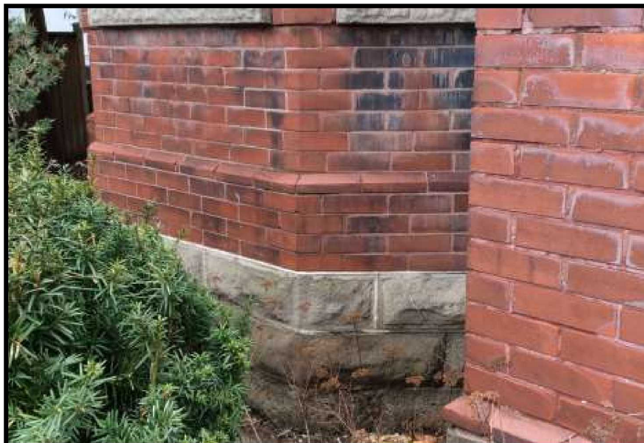
Image 4: Detail of Cut-stone Foundation (Photo taken on April 7, 2016; Facing West)
