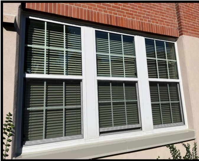
Existing windows - aluminum framed double-glazed fixed and hung window types with simulated muntins, c. 2005.
