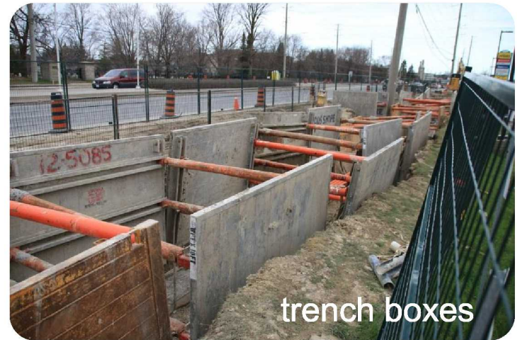
placing trench boxes
