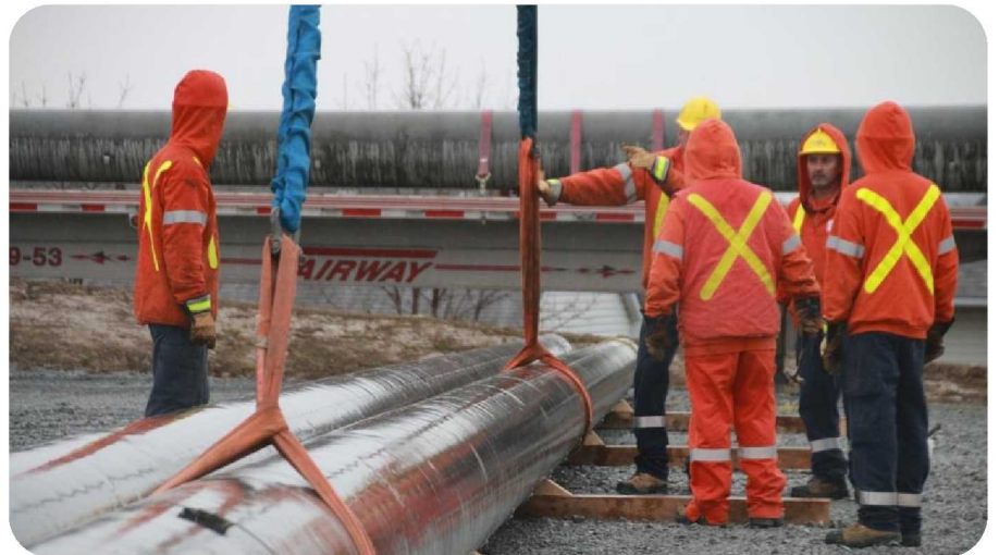
First delivery of 100 foot hydro poles, weighing ~20,000 lbs each
