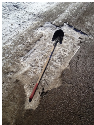
Example of core assets with condition defects: winter freeze and thaw damage.
