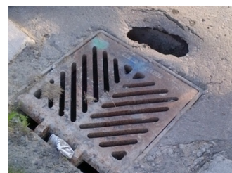
Example of core assets with condition defects: drainage damage caused by a broken pipe.
