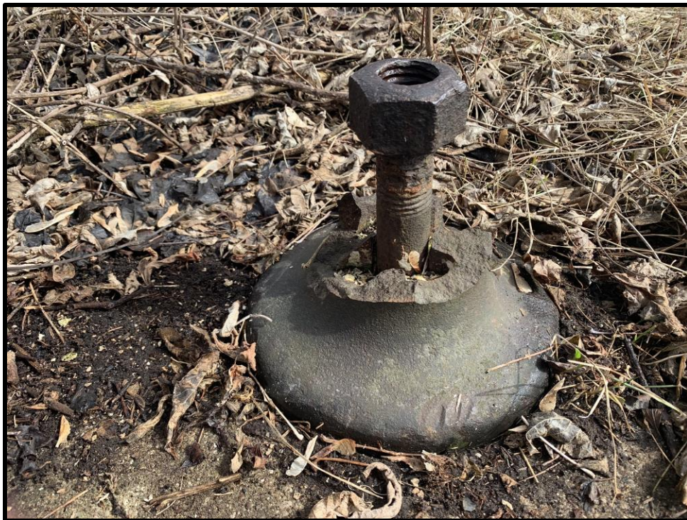
Image 16: Dock cleat bolt without encasement (Photo taken on March 11, 2020)
