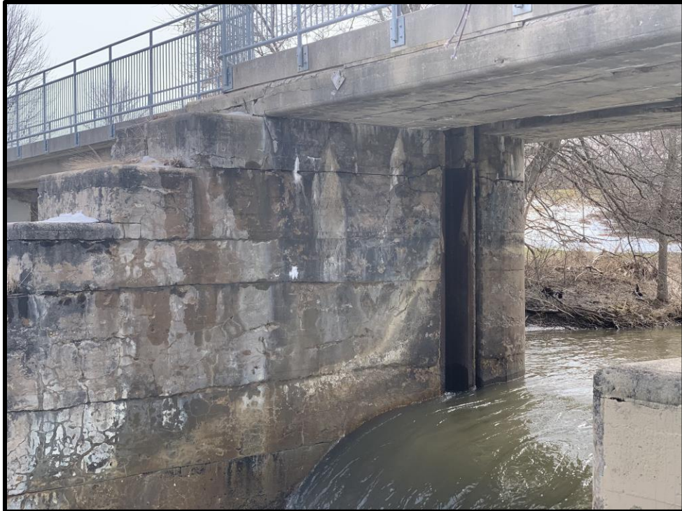
Image 6: Detail of auxiliary spillway (Photo taken on March 11, 2020; Facing East)
