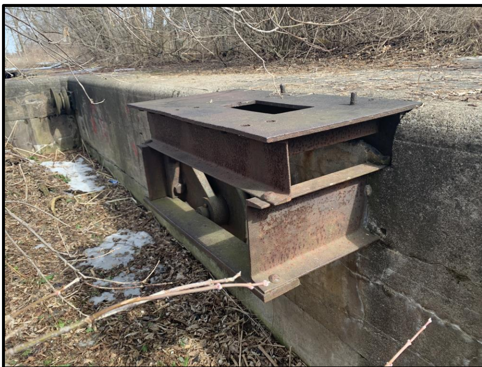
Image 17: Pulley system south side of Lock 3 (Photo taken on March 11, 2020: Facing Northeast)
