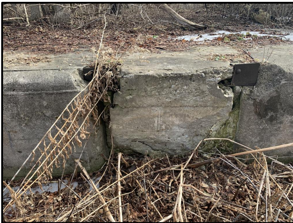
Image 15: Detail of board marks in concrete of Lock 3 (Photo taken on March 11, 2020: Facing West)
