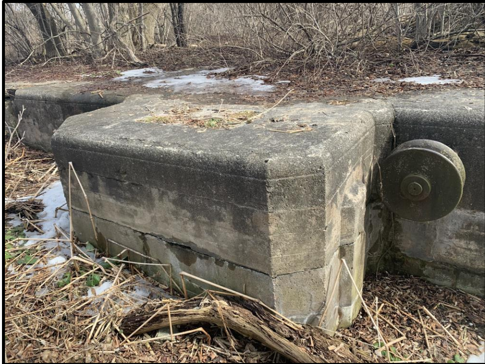
Image 18: Detail of pulley system south side of Lock 3 (Photo taken on March 11, 2020: Facing East)
