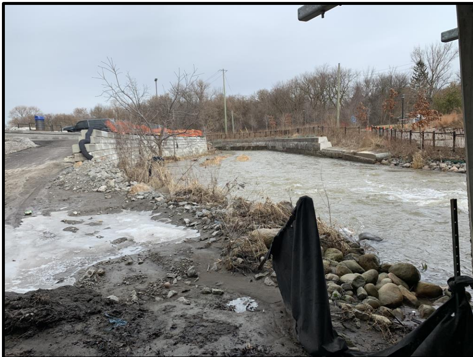
Image 33: Original poured-in-place concrete canal east wall with recent stepped cuts (Photo taken on March 11, 2020; Facing Northeast)
