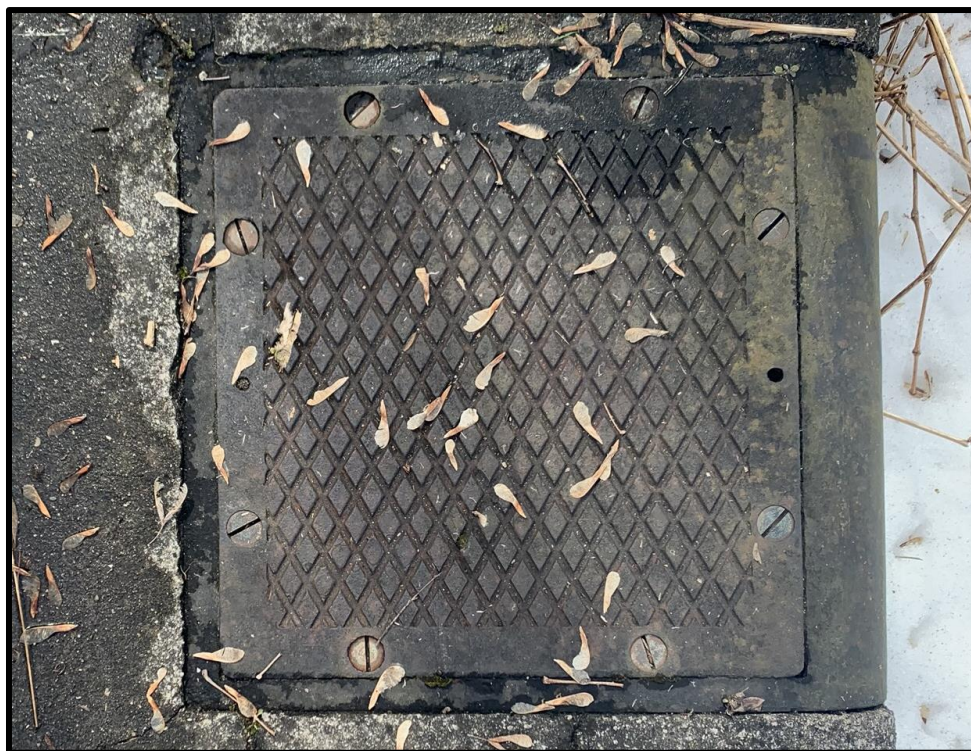
Image 13: Access panel to drain lock chamber of Lock 3 (Photo taken on March 11, 2020)
