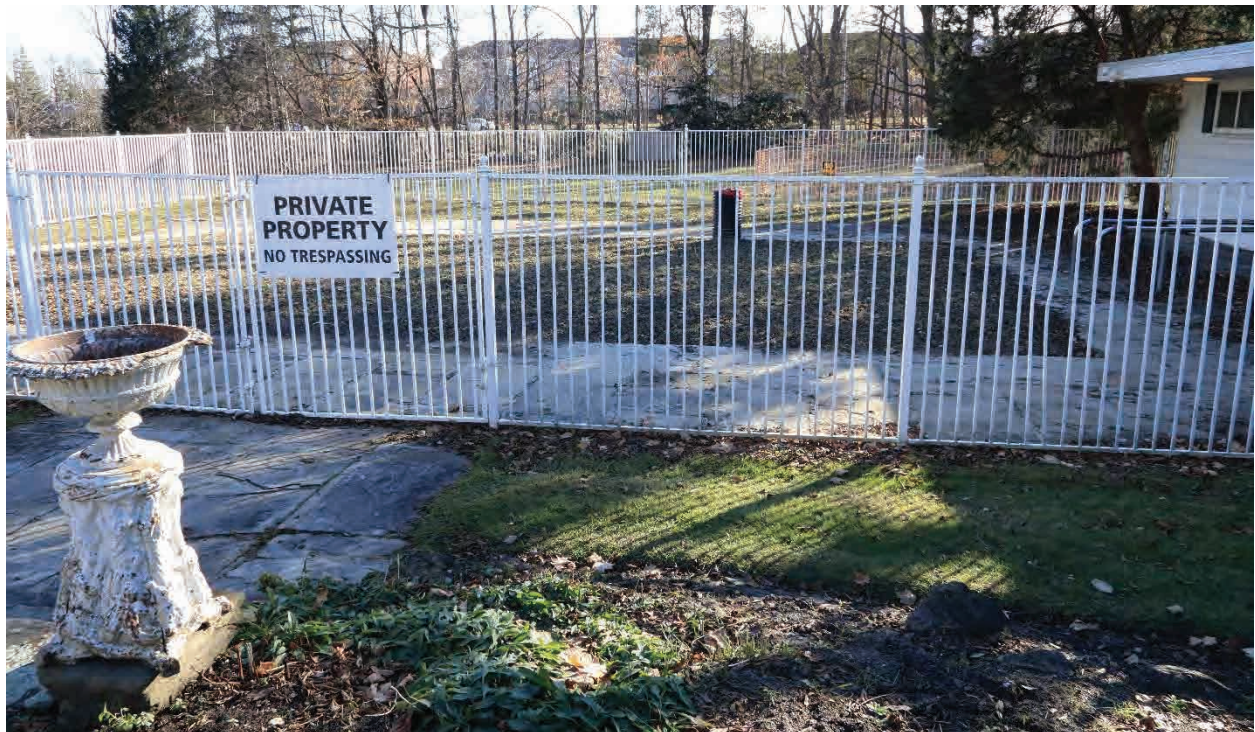
Image 6: South view of the former pool with the existing pool house on the right.
