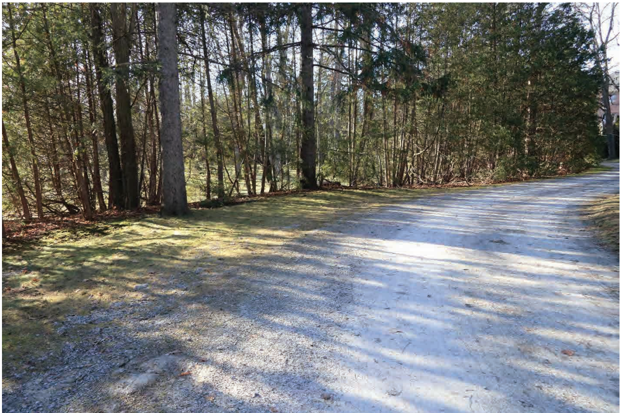
Image 12: Northwest view along gravel drive showing slight cut bank on the right.
