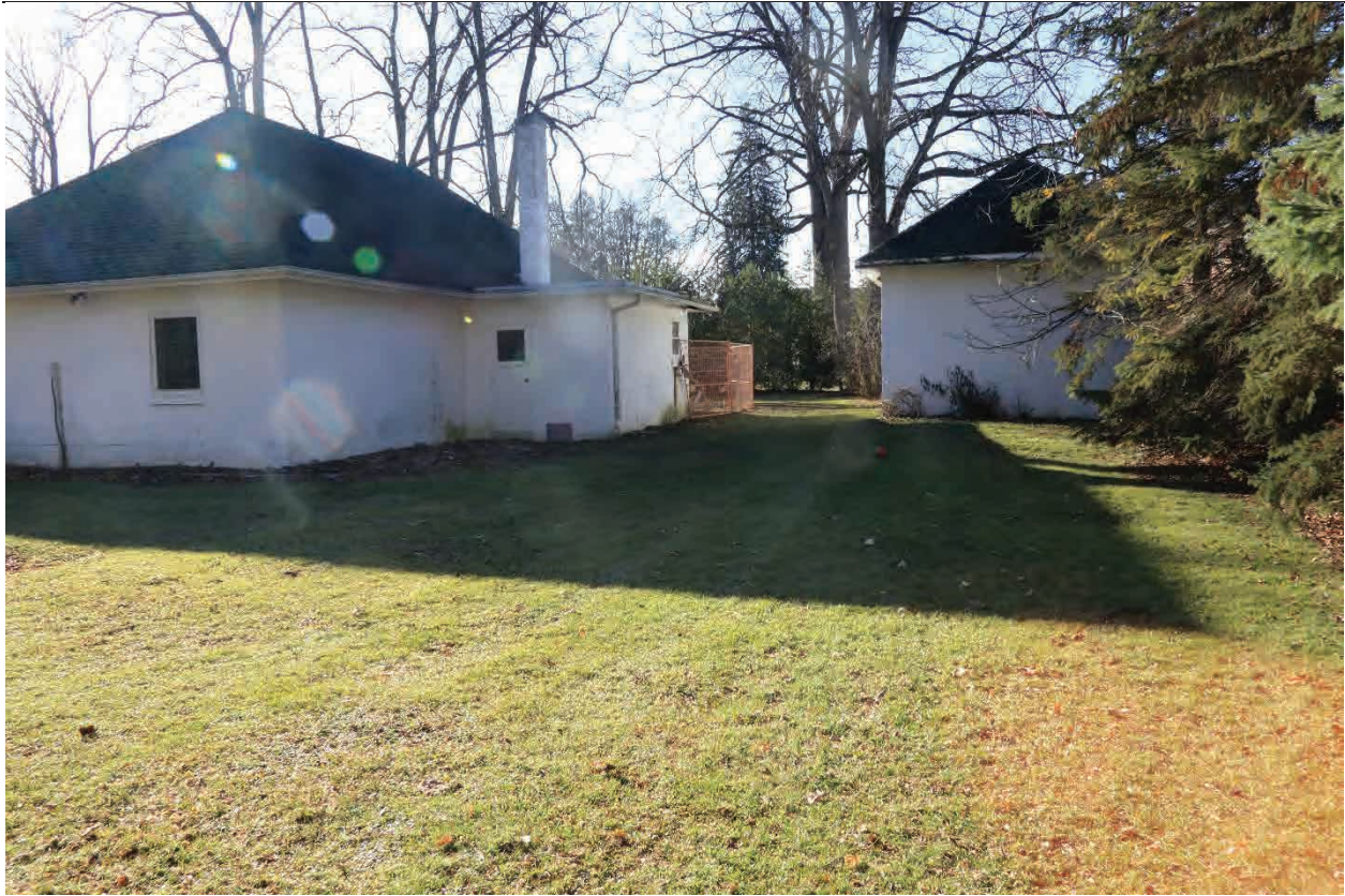
Image 5: West view of the garage (left) and shed (right).
