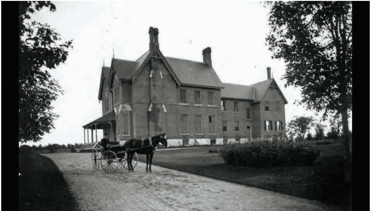
Image 1: South-facing view towards the northeast corner of Mulock house in the early 1900s (NewmarketToday.ca 2018).
