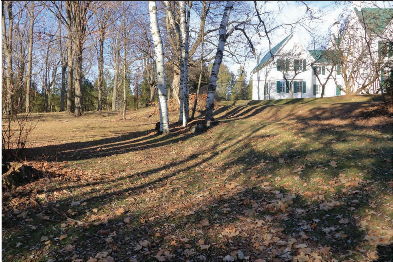
Image 9: North view of west (original) section of the house and terraced landscape in the foreground.
