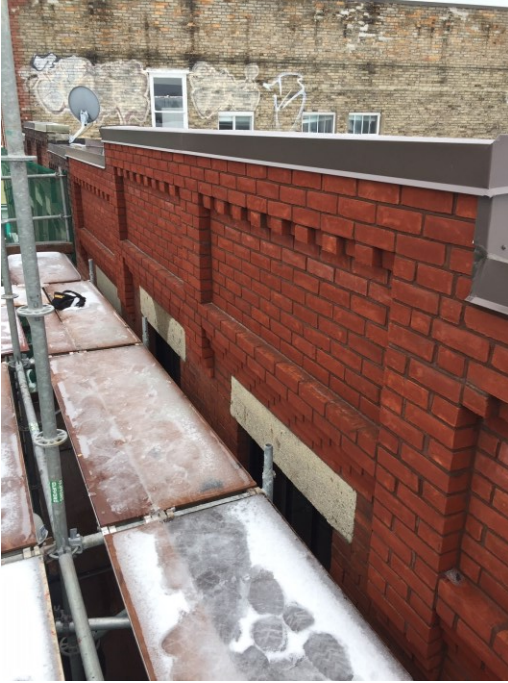
Photo 4: Restored parapet at 194 Main Street
