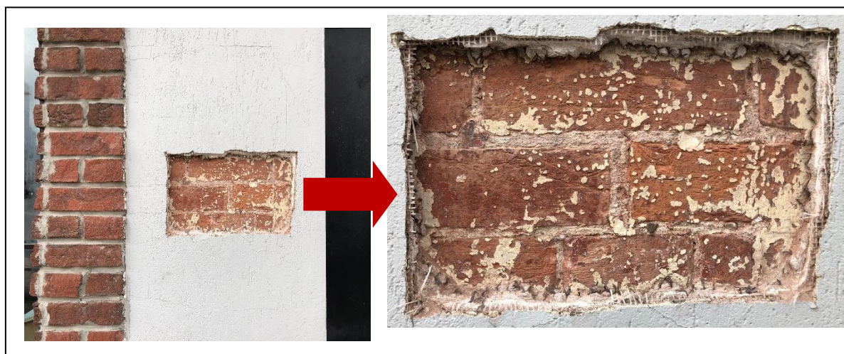
Figure 7.4 Removal of Existing Stucco – sample area. [Source: CSpace Architecture]
