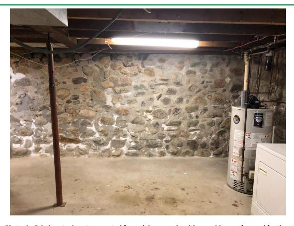
Photo 4 - Existing steel post supported from slab-on-grade with no evidence of spread footing.
