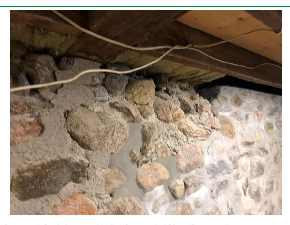
Photo 1 - Existing field-stone rubble foundation wall with loss of mortar and loose stone at top of foundation wall.
