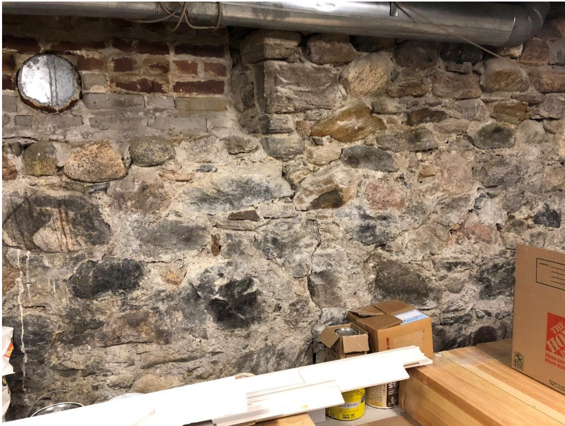
Photo 2 - Existing field-stone rubble foundation wall with evidence of efflorescence stains and vertical crack extending from previous window opening.
