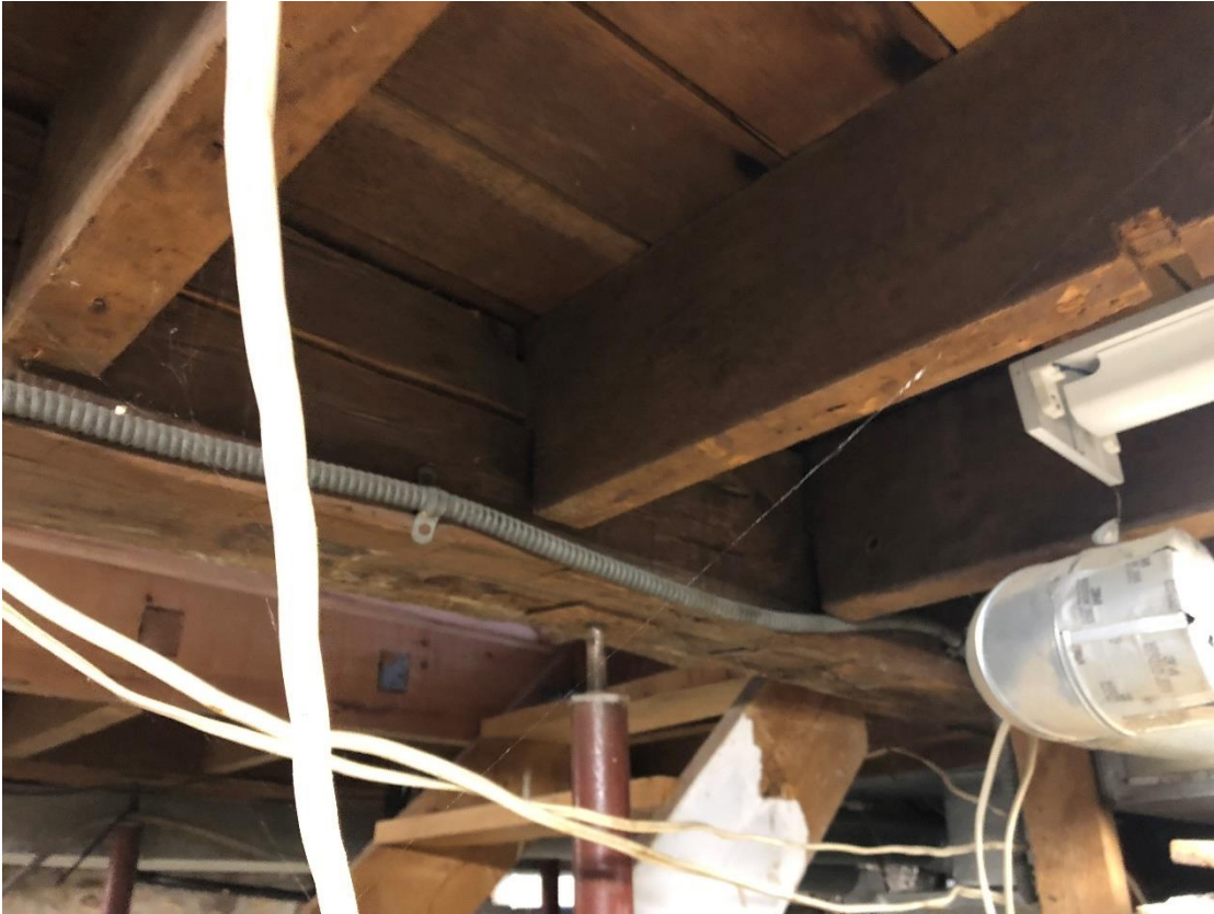
Photo 3 - Existing framing for ground floor and mortise and tenon joint into main structural beam.
