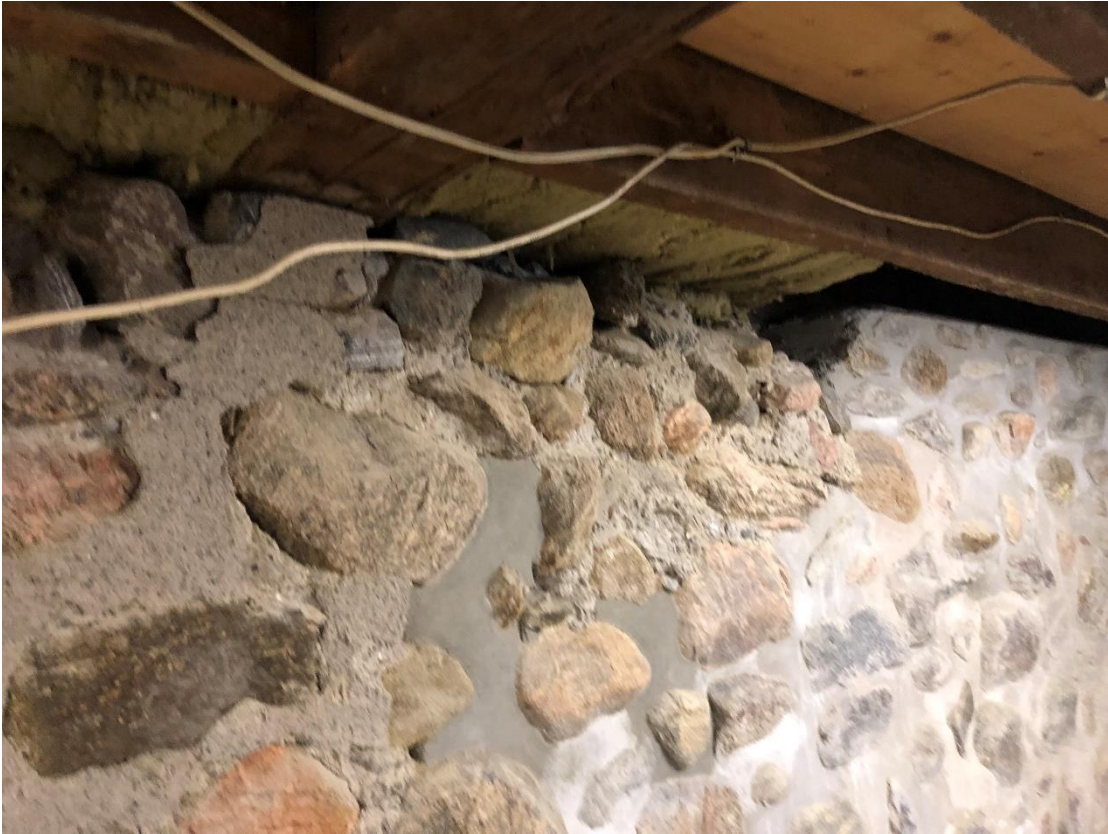
Photo 1 - Existing field-stone rubble foundation wall with loss of mortar and loose stone at top of foundation wall.
