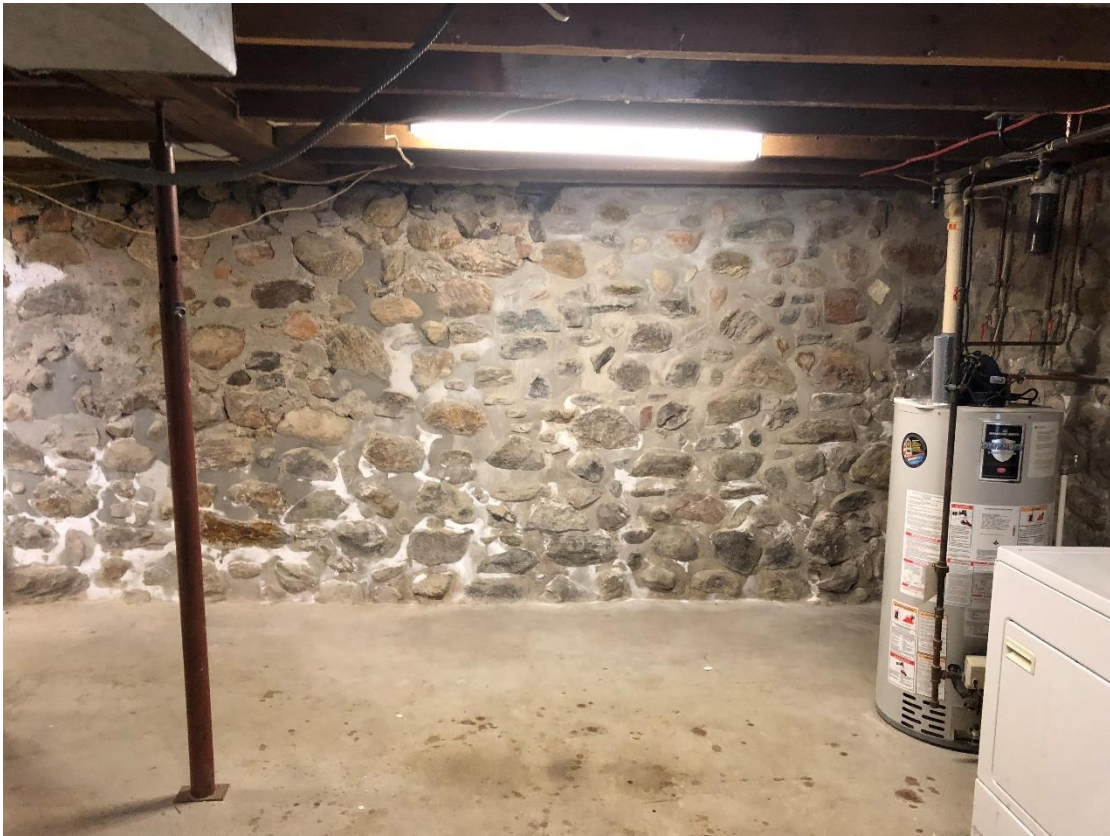
Photo 4 - Existing steel post supported from slab-on-grade with no evidence of spread footing.
